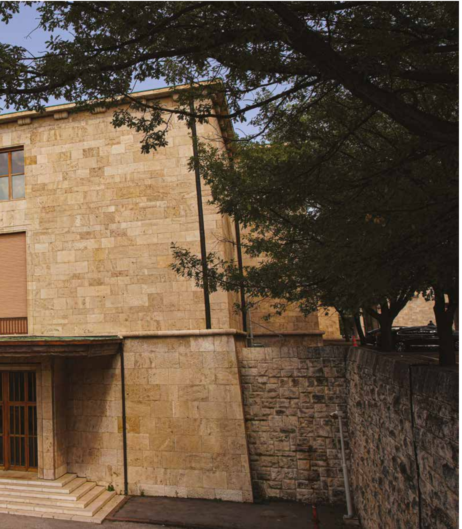
The Ceremonial Hall, West Façade
