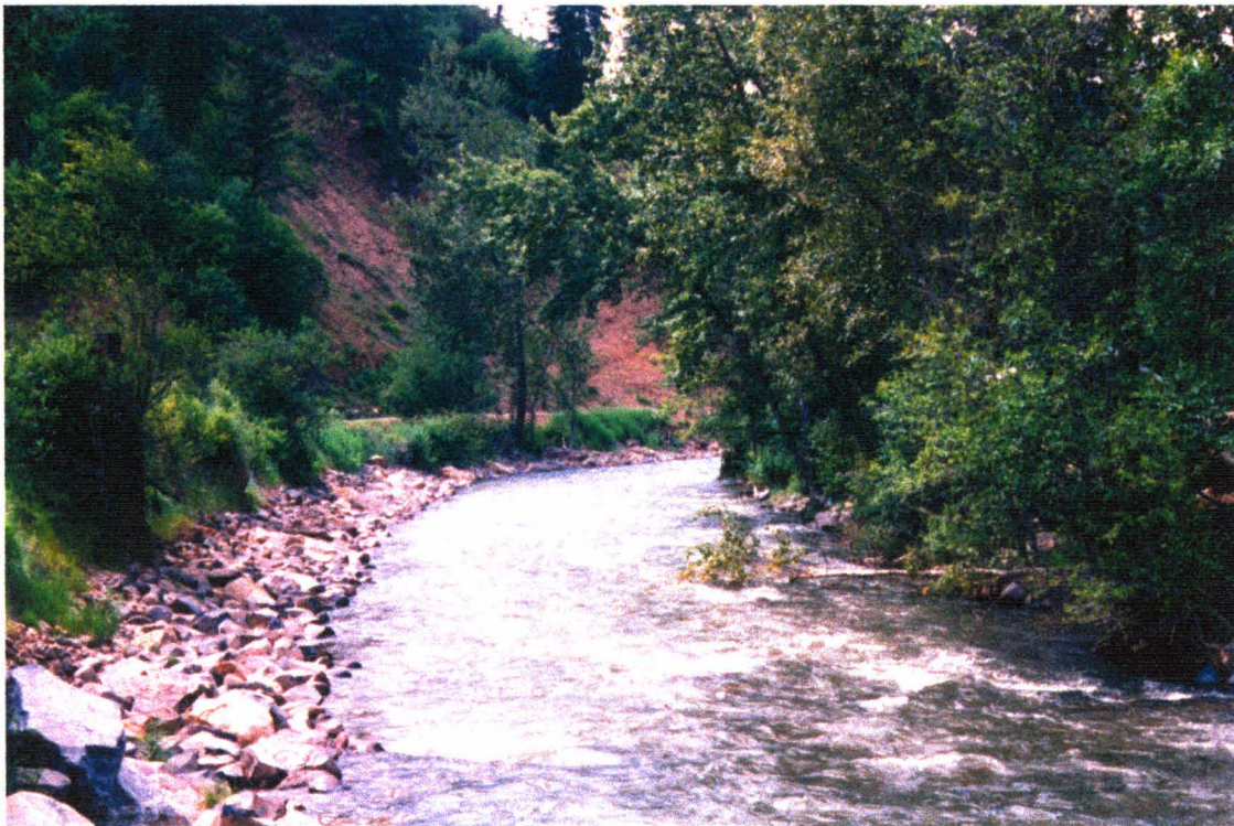
Figure 11: Photograph showing landslide site 23. (Notice mitigation of stream channel.)
