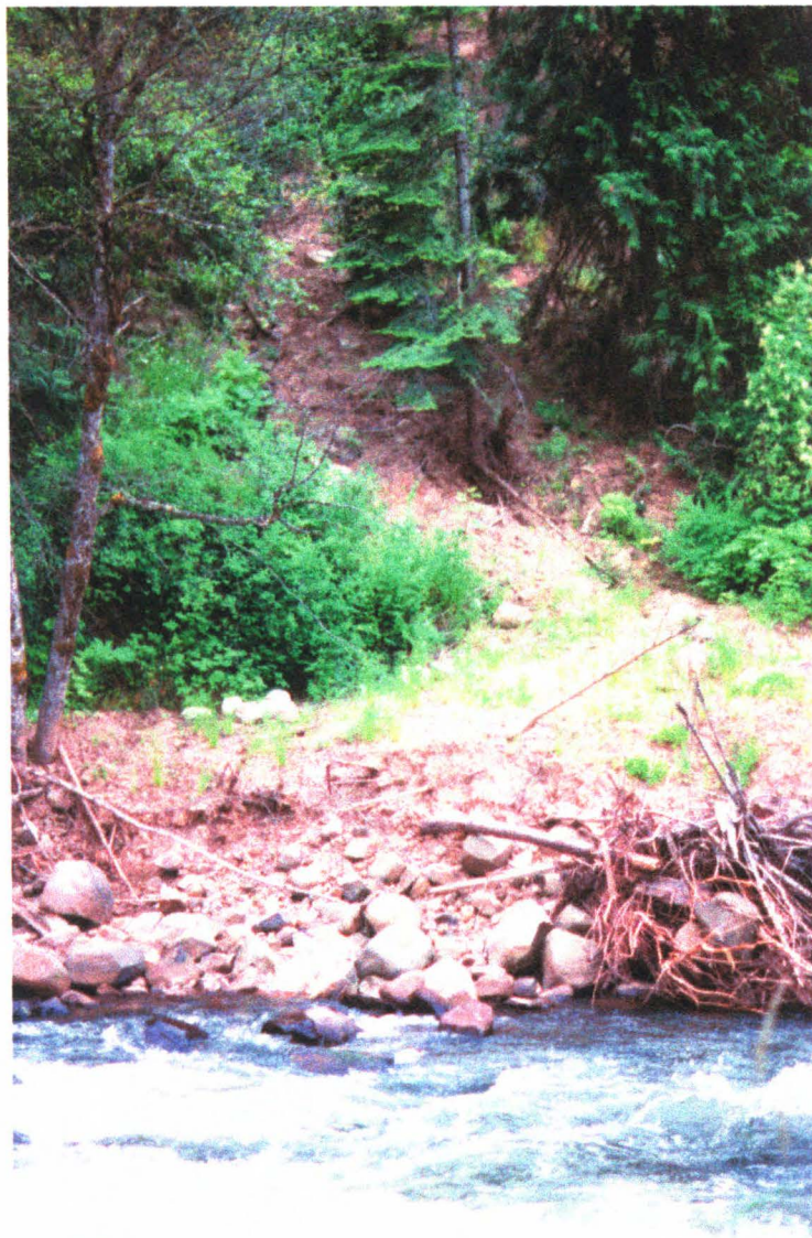
Figure 17: Photograph of Landslide at site 31.
