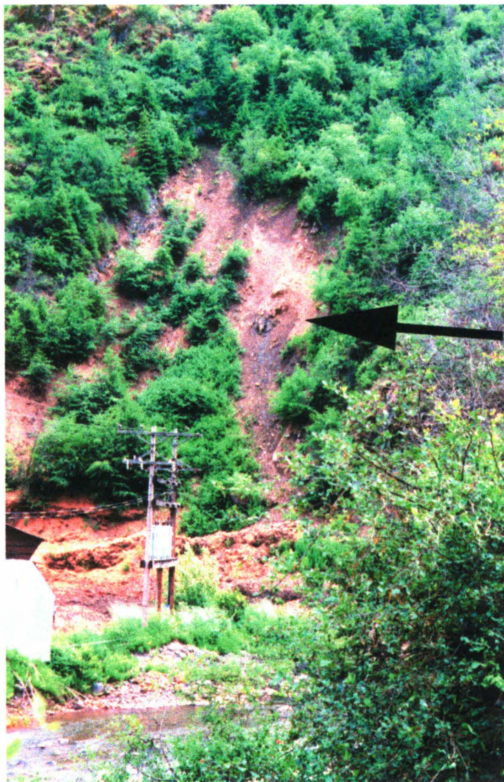
Figure 14: Photograph of landslide at site 27. Arrow indicates location of springs.
