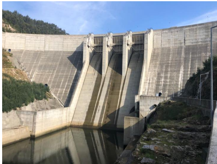
Fig. 3 – Downstream view of Ribeiradio dam
