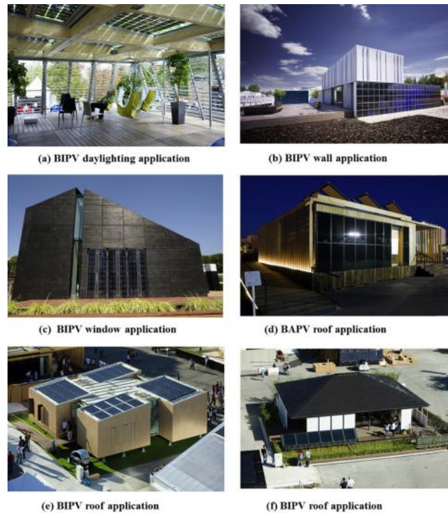
Figure 3 Applications of panels in a building [10]
