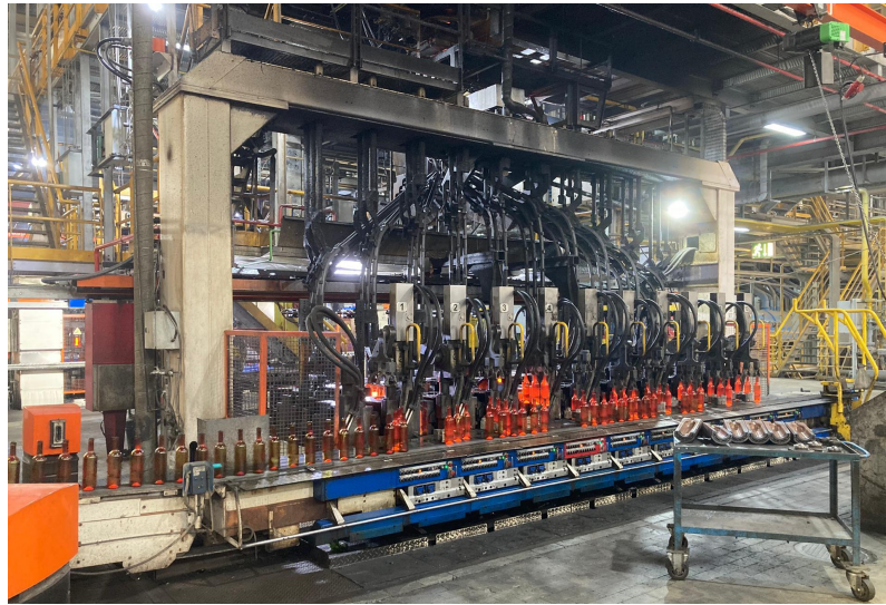
Figure 3.4: Triple gob IS Machine at the line 53 in the Avintes plant
