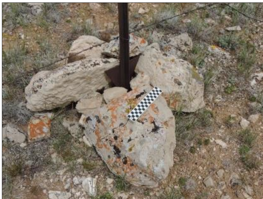
Figure 2.3. Recent NPS cairn construction supporting fence post.
