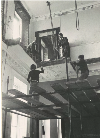
Figure 3.6: No. 15 Dawson Street, Dublin, first-floor ceiling during removal in February 1977.
