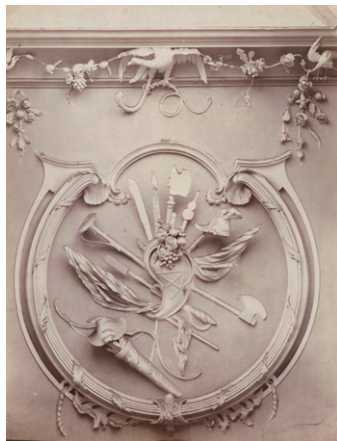
Figure 3.18: No. 129 St Stephen's Green, Dublin, built mid-eighteenth century, demolished 1986. Carved timber and plasterwork on staircase wall, from Georgian Society Records , vol. II (Dublin: 1910).
