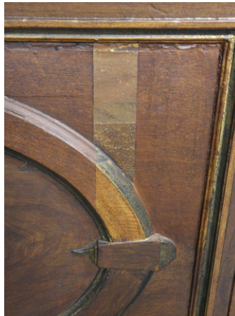
Figure 2.27: Ham House, reveals of past wood-graining campaigns.
