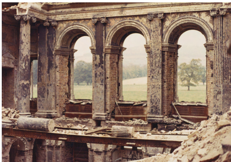
Figure 5.12: Saloon, Powerscourt, County Wicklow in the aftermath of the fire in 1974.
