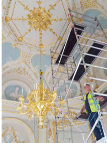
Figure 6.13: Installation of chandelier at Orleans House Gallery, Twickenham, London.
