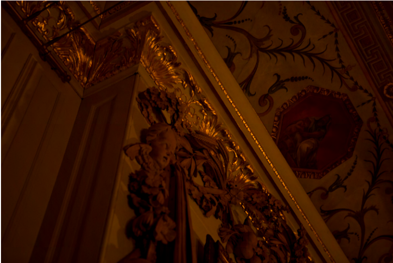
Figure 4.11: The effects of candlelight on carving, gilding and painting at Kensington Palace. The gilding and white paint replicate elements installed by William Kent in 1725. The carvings are by Grinling Gibbons.
