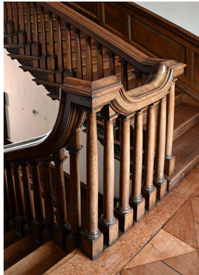
Figure 11.16: Staircase at Russborough, County Wicklow.
