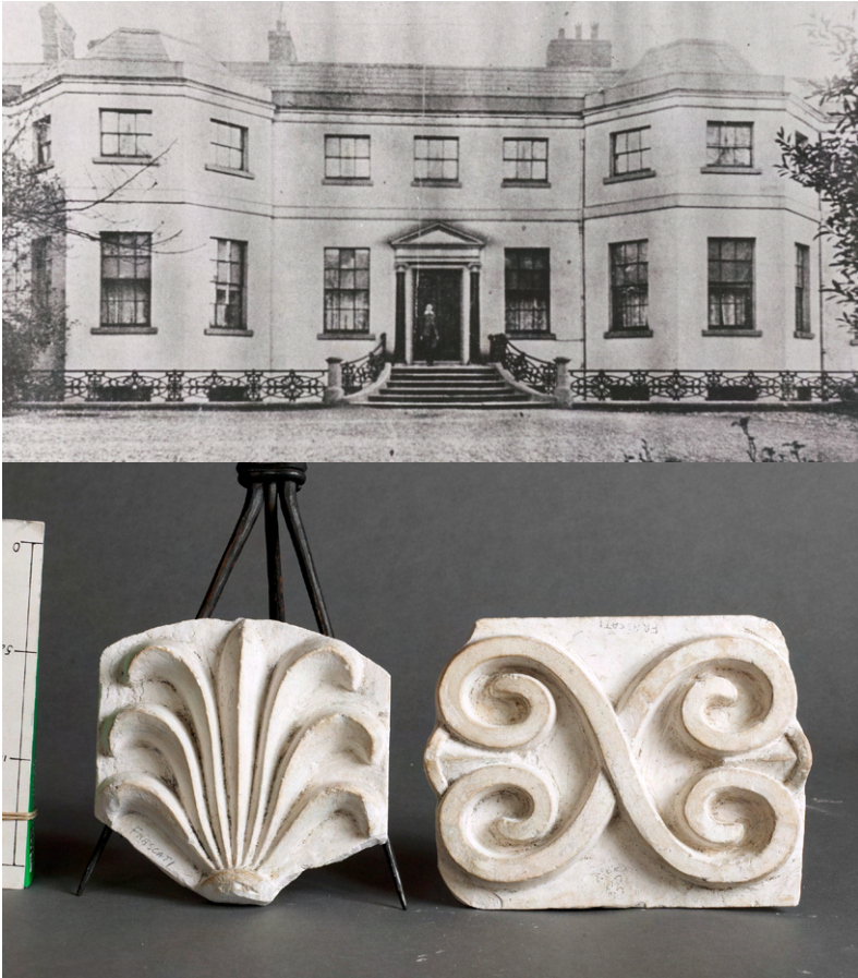
Figure 3.4: (a) Frescati House, Blackrock, County Dublin, built 1739, demolished 1983. Photograph from The Lady of the House (Christmas, 1908). Courtesy of the Irish Architectural Archive; (b) Plaster anthemion and piece of strapwork, Frescati House, Blackrock, County Dublin.
