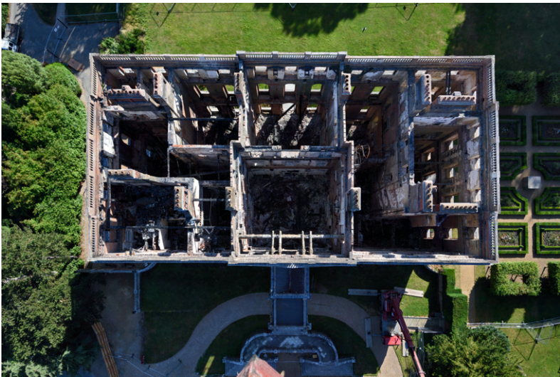
Figure 1.24: Clandon Park, looking into the gutted house in the days after the fire.
