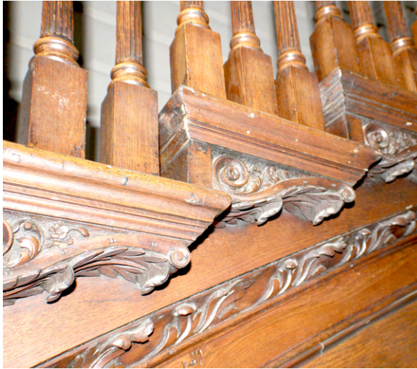
Figure 11.5: Bracketed tread ends, staircase of the Old Library, Trinity College Library, Dublin.
