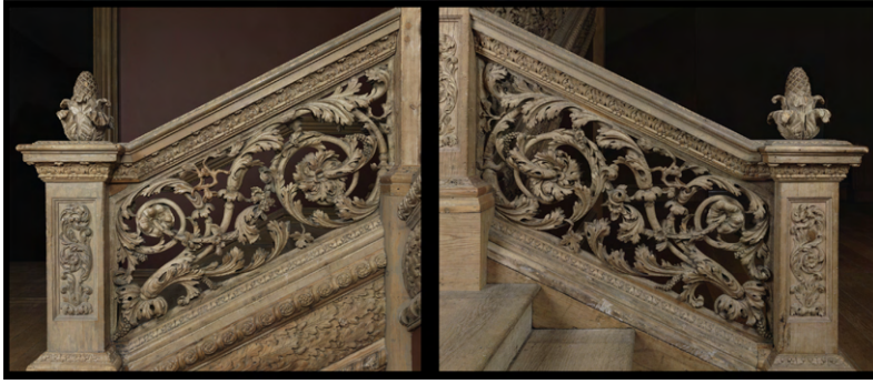
Figure 2.2: Balustrade of bottom short flight, Cassiobury Park staircase. Exterior side (left); interior side (right).
