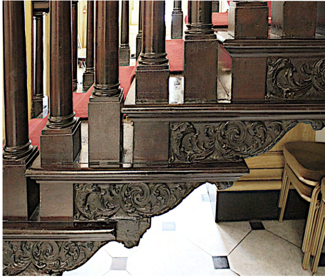
Figure 11.14: Staircase at No. 85 St Stephen's Green, Dublin.
