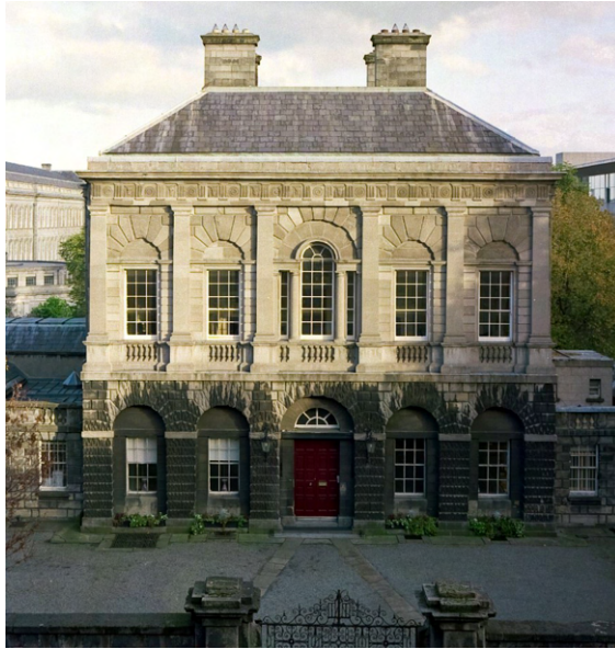
Figure 8.13: Ardraccan limestone, Provost's House, Trinity College Dublin. The icicle rustication on the ground floor has allowed for the build-up of soot and gypsum while the upper story, being plain ashlar, remains cleaner. Photograph by Stephen Farrell.
