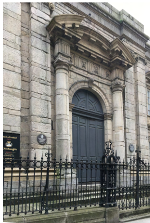
Figure 8.5: St Werburgh’s Church, Dublin. Entrance façade with Calp limestone plinth and worked Scrabo sandstone laid in a pattern of courses of unequal size.
