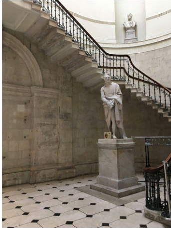
Figure 8.10: Portland stone, interior, former Royal Exchange, Dublin. It is possible that the Portland floor with insets of Kilkenny black marble was restored in the early twentieth century.
