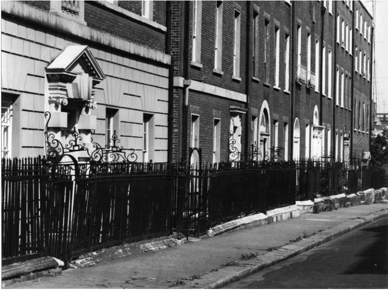
Figure 3.28: Wrought-iron railings, Nos. 3–9 Henrietta Street Dublin, built circa 1730–56.
