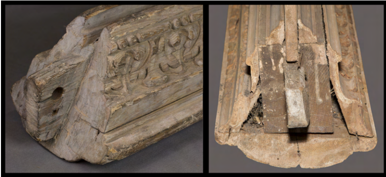
Figure 2.28: Handrails from Cassiobury (left) and Eyrecourt staircases (right), showing the effects of the chemical stripping.
