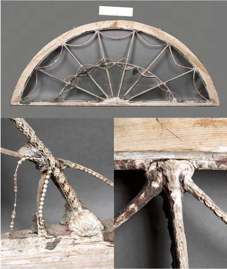
Figure 3.25: (a–c) Fanlight, gesso on timber, with ram’s head ornament, Lower Leeson Street, Dublin, late eighteenth century.
