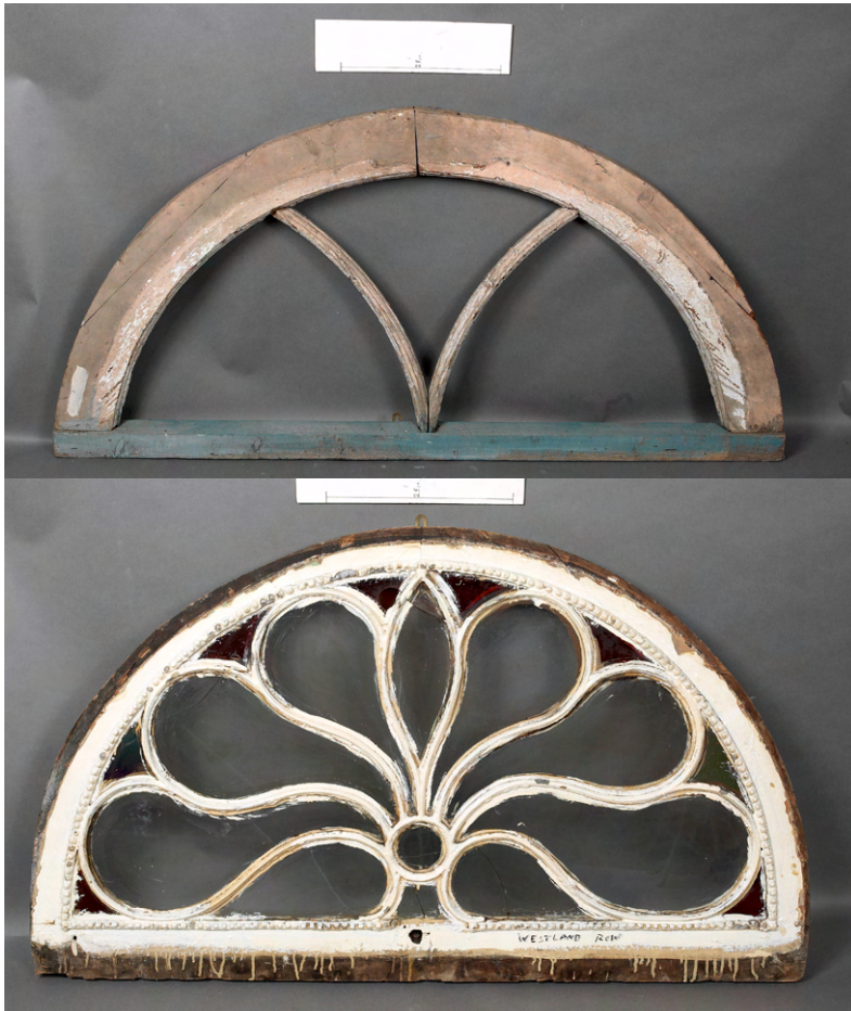
Figure 3.24: Timber fanlights: (a) Fownes Street, Dublin, circa 1750; (b) Westland Row, Dublin, late eighteenth century.
