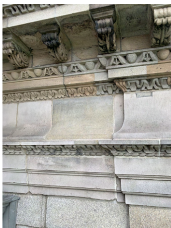
Figure 8.4: Old Library, Trinity College Dublin. Cornice-level carvings in Scrabo sandstone (top), Calp limestone (middle) and ashlar granite (bottom). Compared with contemporary carvings in Portland stone in Dublin these are rather crude. Some of the sandstone has been replaced with moulded mortar.
