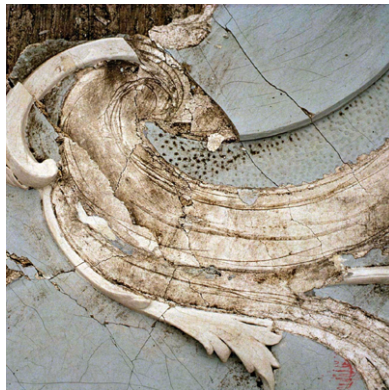
Figure 9.8: Early eighteenth-century plasterwork where sections of the applied ornament have fallen away to reveal the scored surface underneath in the dirty white central section. Small parts of the modelled leaf have survived around the edges of the exposed scoring.
