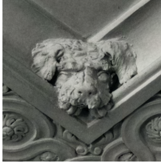
Figure 1.21: Clandon Park, the Library ceiling, showing its simple cove, repetitive guilloche and hand-modelled terrier.
