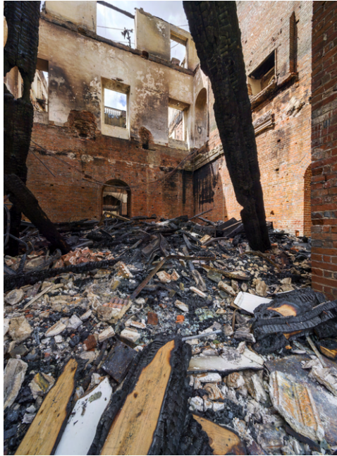
Figure 1.25: Clandon Park, the Saloon, showing sections of the surviving frieze and plaster fragments in the debris.
