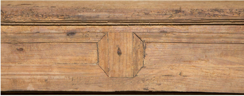
Figure 2.26: Detail of Eyrecourt staircase step.
