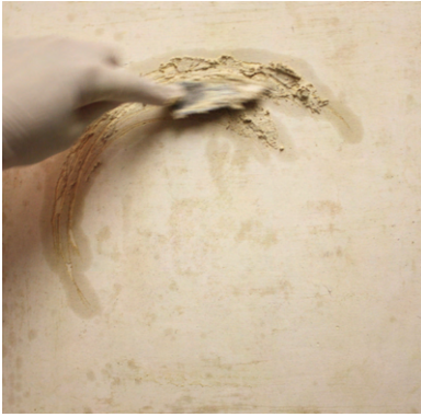
Figure 9.10: Lime-plaster modelling demonstration: application of coarse 'stuff'.
