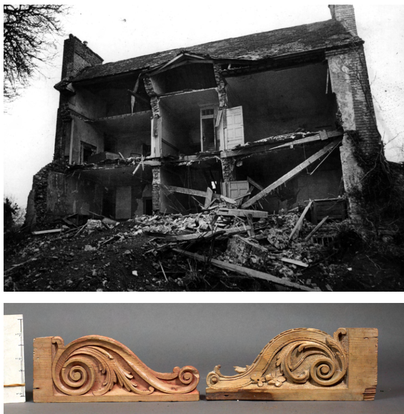
Figure 3.13: (a) Allenton House, Tallaght, County Dublin, showing façade removed on New Year's Day, 1983; (b) carved timber bracket, Allenton House (left).
