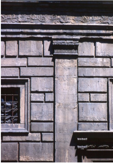
Figure 7.2: Palazzo Rucellai, Florence, L.B. Alberti, 1447 onwards, drafted masonry of façade.
