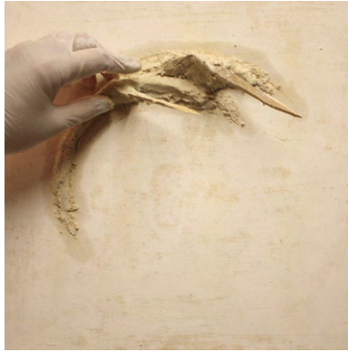
Figure 9.13: Lime-plaster modelling demonstration: addition of armature.
