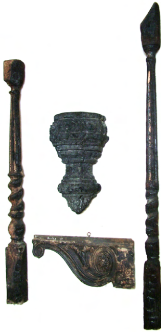
Figure 3.9: Charred timber balusters, Kilmacurragh, County Wicklow.
