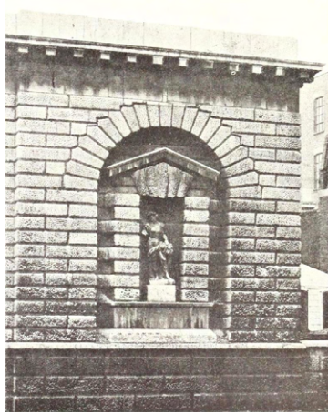
Figure 7.8: Newgate Prison, London, George Dance, 1770–80, detail of façade. From A.E. Richardson, Monumental Classic Architecture in Great Britain and Ireland during the XVIIIth and XIXth Centuries . London: Batsford, 1914, p. 29, Figure 32.
