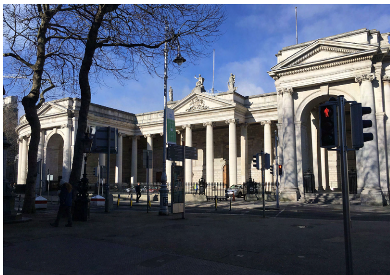
Figure 8.1: Former Parliament House, now Bank of Ireland, College Green, Dublin. Portland stone colonnade with granite walling.
