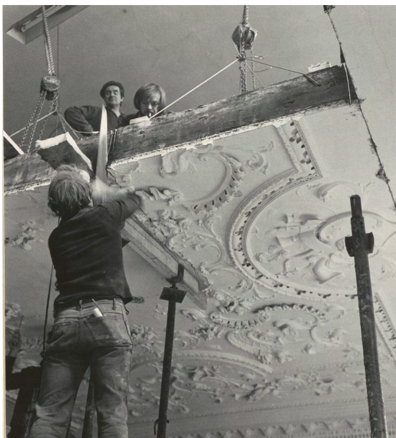
Figure 3.17: No. 15 Dawson Street, Dublin, first-floor ceiling during removal in December 1977.
