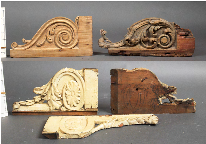
Figure 3.14: (a) and (b) Eighteenth-century timber brackets, No. 127 St Stephen's Green, showing sketch on reverse.
