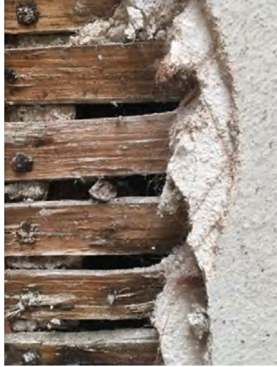
Figure 1.30: Layers revealed by the fire, including the softwood laths and three layers of plaster.
