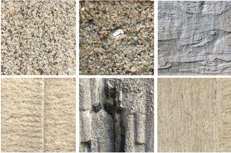
Figure 8.3: (a) Granite of Baltyboys/Blessington type at the former Parliament House, Dublin, comprising equigrained sized interlocking crystals of quartz, feldspar and mica providing a pale-grey colour; (b) Three Rock Mountain granite with characteristic large mica crystals set into smaller crystals of quartz and felspar (detail from Dublin Castle wall); (c) Calp limestone with fine-bedded laminations of limy sediment with intercalations of more muddy horizons, all traversed by thin vertical white veins of calcite (detail from Old Library, Trinity College Dublin); (d) Scrabo sandstone comprising coarse quartz sand grains – drafted margin of stone seen at centre left (detail from Treasury Building, Dublin Castle); (e) Ardraccan limestone containing fossil crinoid stems top right and icicle rustication (detail from Provost’s House, Trinity College Dublin.); (f) Portland stone with fine oolitic grains and some fragmented shelly fragments and tooling marks (detail from Public Theatre [Examination Hall] column, Trinity College Dublin). Width of field of view 10 cm for each.
