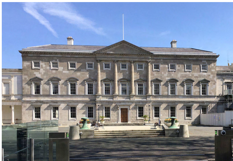
Figure 8.12: Ardbraccan limestone, Leinster House, Dublin. The pale ashlar inserts are in Lecarrow limestone from County Roscommon and date to a recent restoration.
