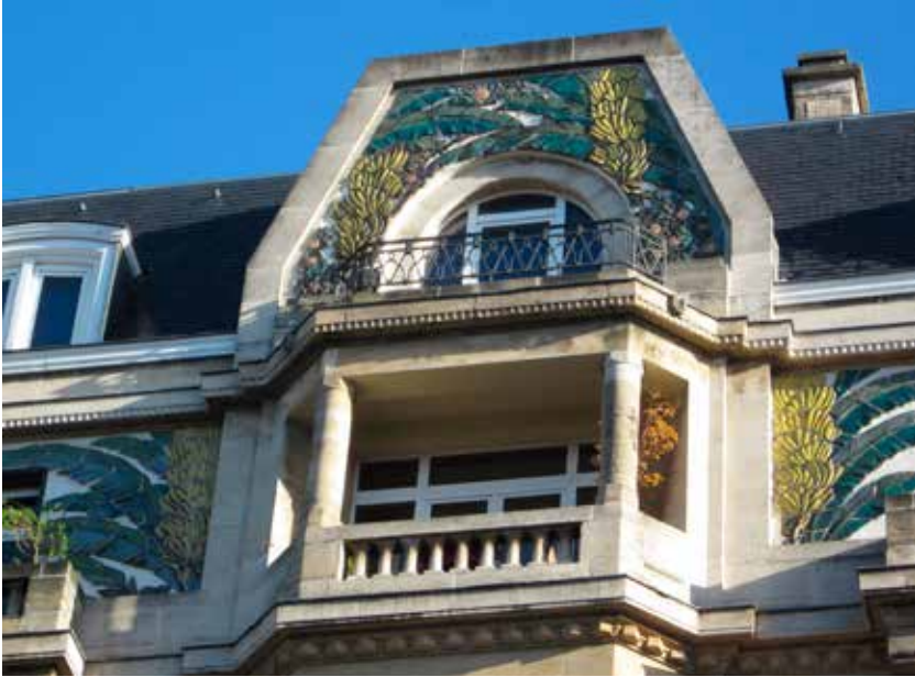
Former G.K.F. building, Brussels, 2013
