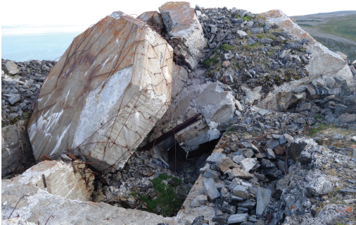
Fig. 3. The exploded carapace of the command and control bunker at Sværholtklubben. Photo: B. Olsen.
