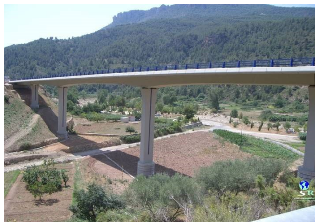
Figure 2. Viaduct in Villahermosa, Spain 2005 (photo by the fourth author).
