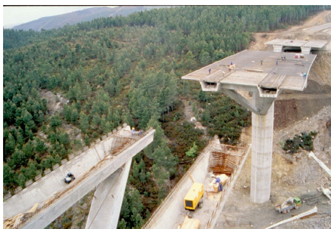
Figure 1. Viaduct over Mente River, Spain 1998. (photo by the second author).
