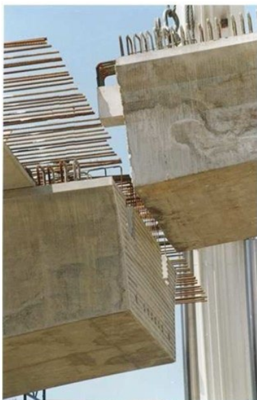
Figure 13. Typical connection detail between beams.
