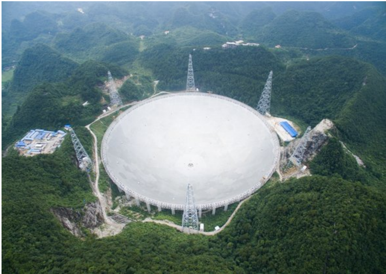
Figure 1.12: The Five hundred meter Aperture Spherical Telescope (FAST) located in China is the largest single dish telescope. Its diameter is 500 m, resulting in a collecting surface of 196 \times 10^3 \text{ m}^2 . (Image credit: VCG/VCG via Getty Images)
