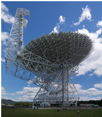
Figure 1.11: The Green Bank Telescope (GBT) located in Virginia, USA, is the largest fully steerable, single dish radio telescope. Its surface is an ellipsoid, measuring 100 by 110 metres, with a collecting surface of 9.3 \times 10^3 m 2 . (Image credit: Wikipedia Commons)
