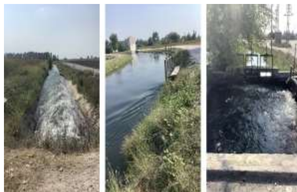
Figure 1 Water supply canals
