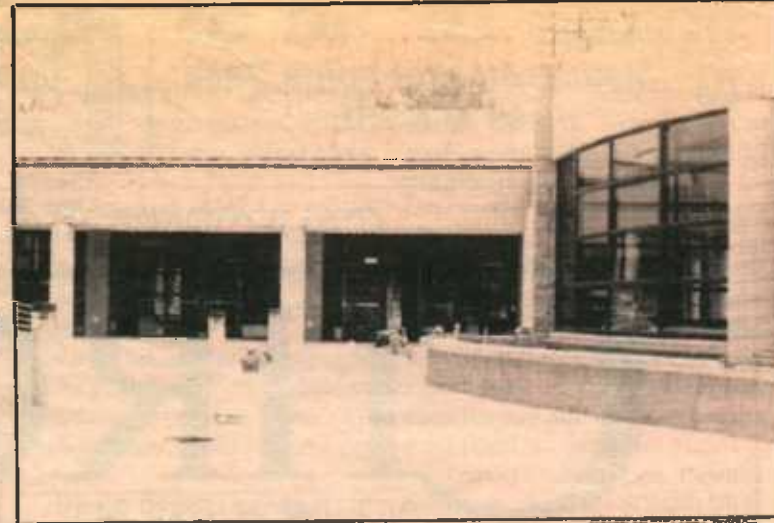
The new student Union building near completion
