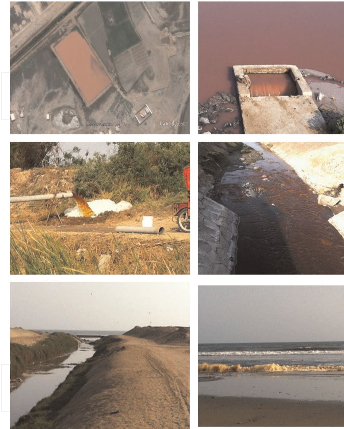
Figure 18. Oxidation lagoon and disposal of treated water in the district municipality of Santa Rosa Lambayeque, Peru (copyright of Reingeniería en Saneamiento ltd).
