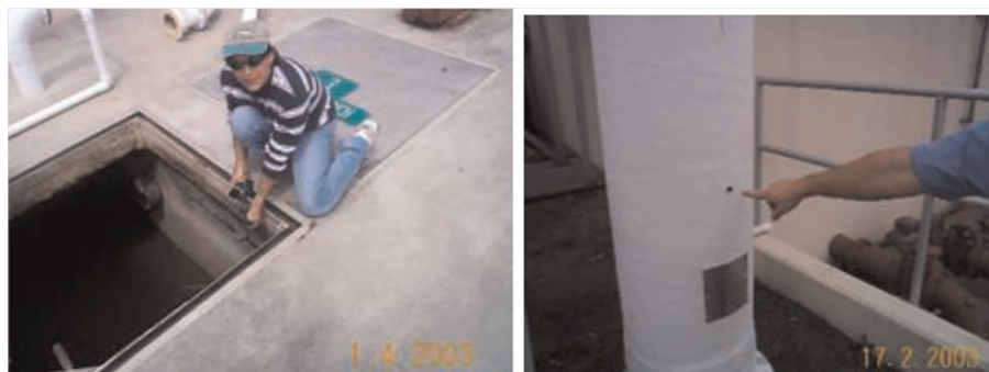
Figure 6. Readings taken in Septage tank (with TRIO 3 permitted authorization).
