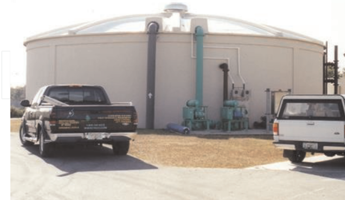
Figure 9. Sludge thickener facility (with TRIO 3 permitted authorization).
