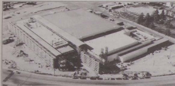
Aerial view of progress on Ontario Convention Center and its 17.5 acres.
