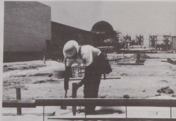
A workman during early phases of construction at Ontario Mills.
