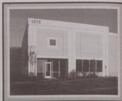
One of the nine brand-new buildings totaling 230,000 sq. ft., recently sold to relocating companies, at West Corona Business Park
