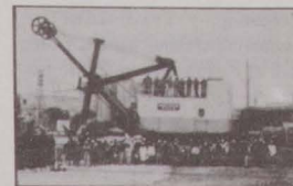
The California Portland Cement plant in Colton
