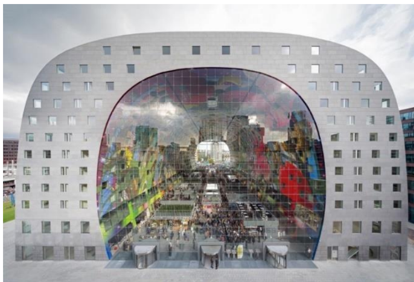
Figura 3. Vista Frontal de Market Hall. Fuente: ArchDaily (2014)
