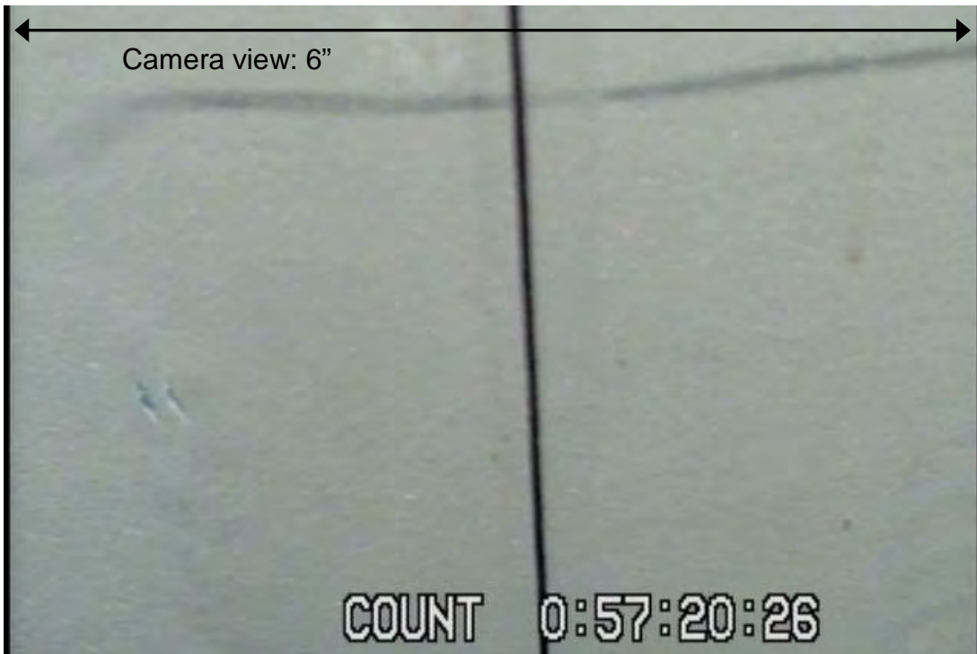
37. Scan 77 coating chips, no discoloration
