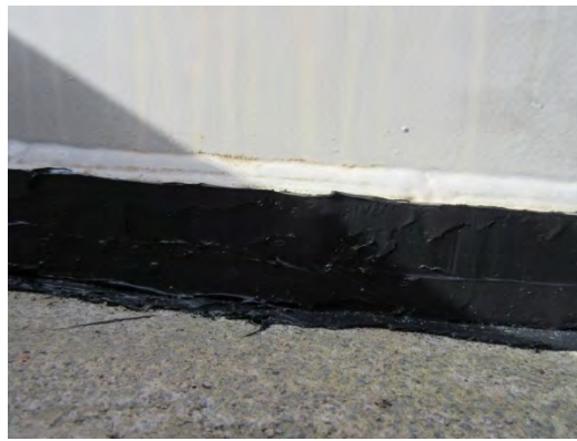
16. Cell 2 Caulking As-Left
