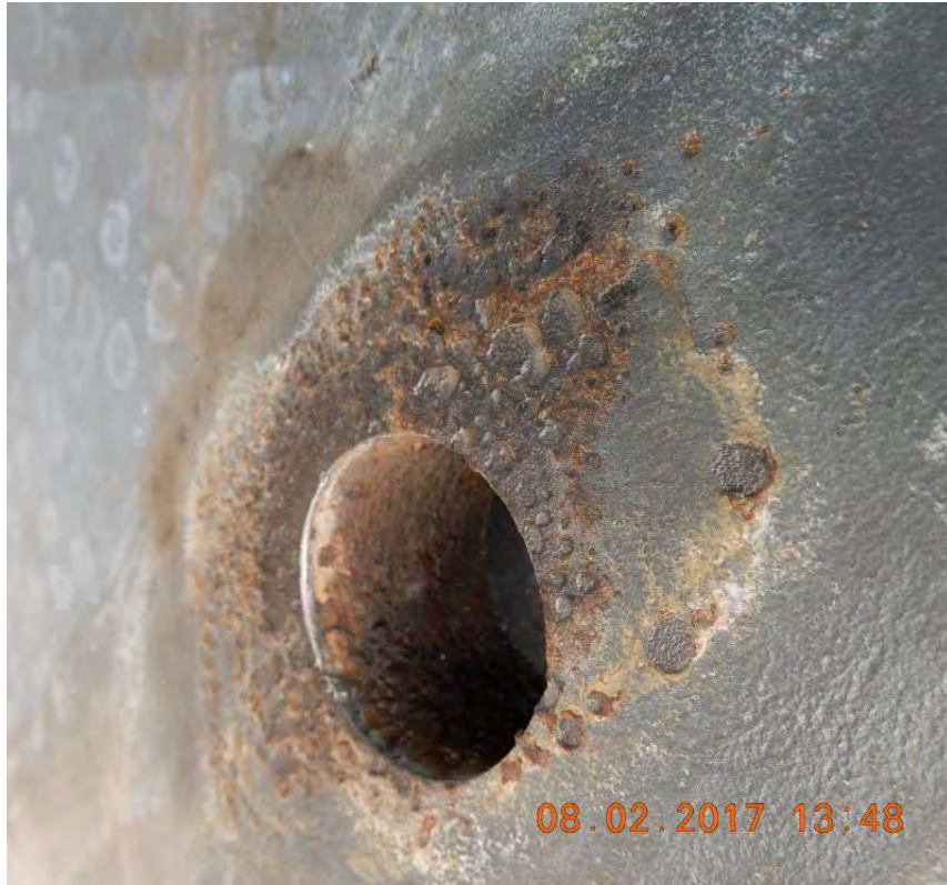
9. Hole #5 after cleaning
