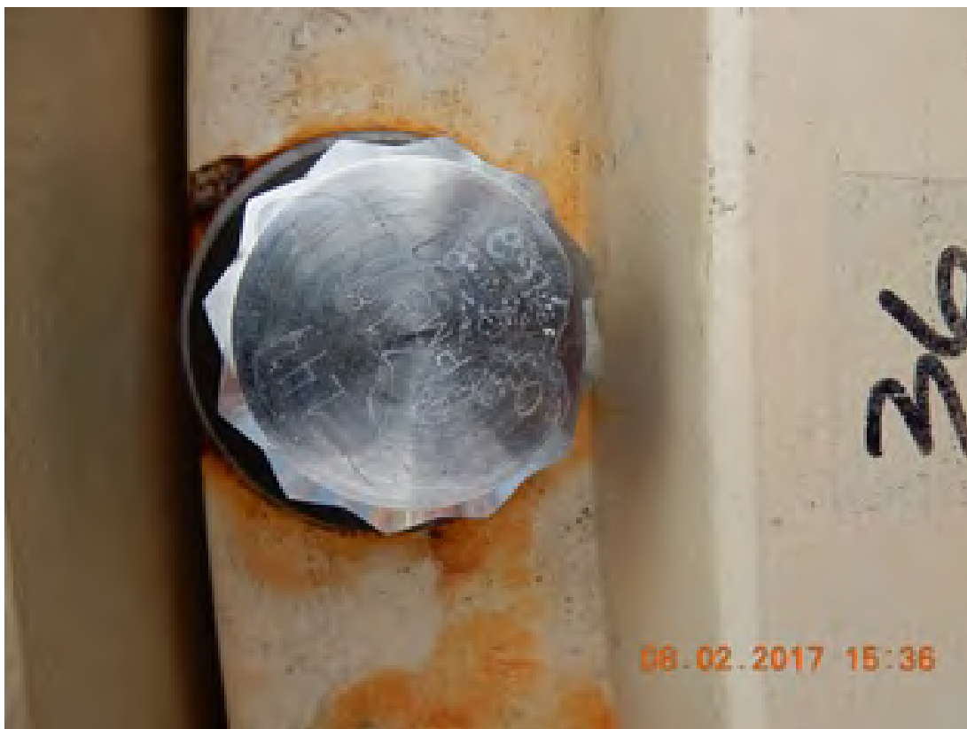
19. Chipped coating under overpack closure lid bolt (at 10 o'clock)
