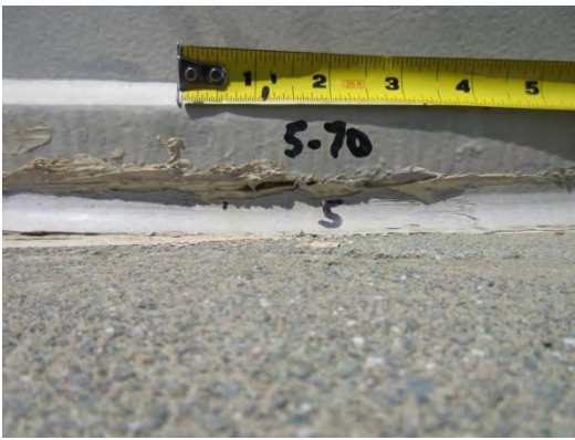
9. Cell 5 Caulking As-Found
