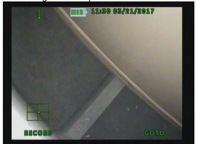
19. Seismic shim and bottom of vault liner
