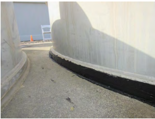
15. Cell 2 Caulking As-Left
