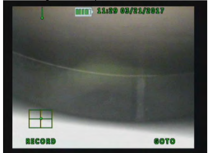
15. Looking down overpack at seismic shim
