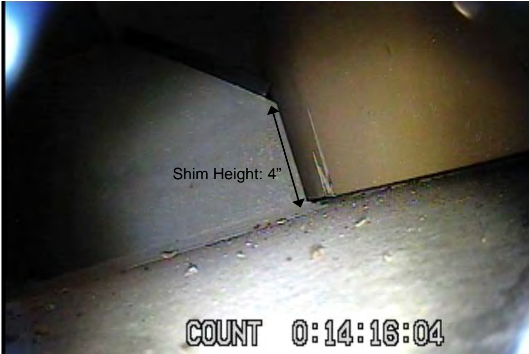
44. Overpack south section coating scrape adjacent to seismic shim
