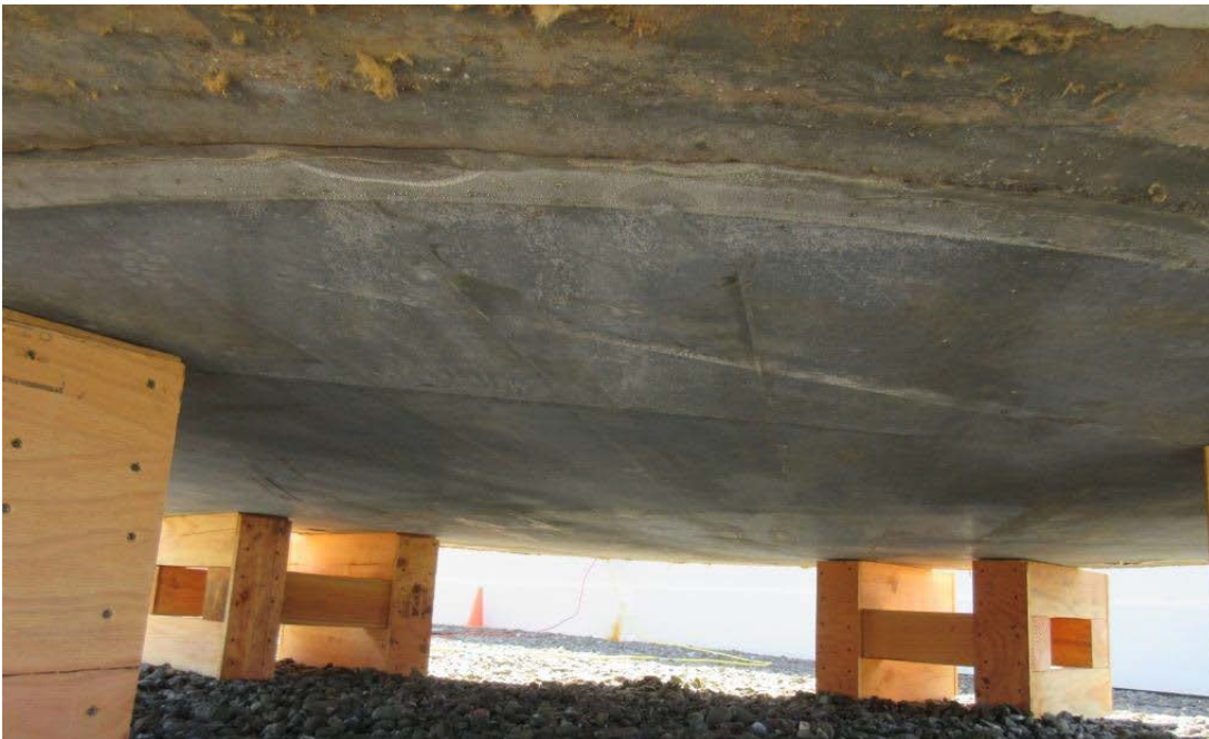
6. Underside of lid general view
