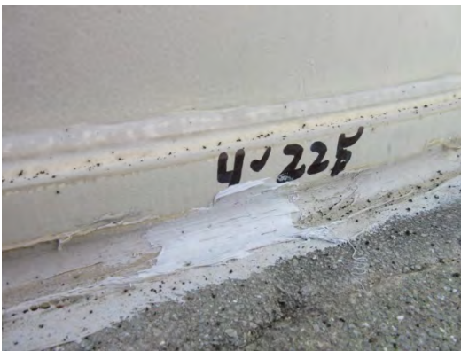
17. Cell 4 Caulking As-Left
