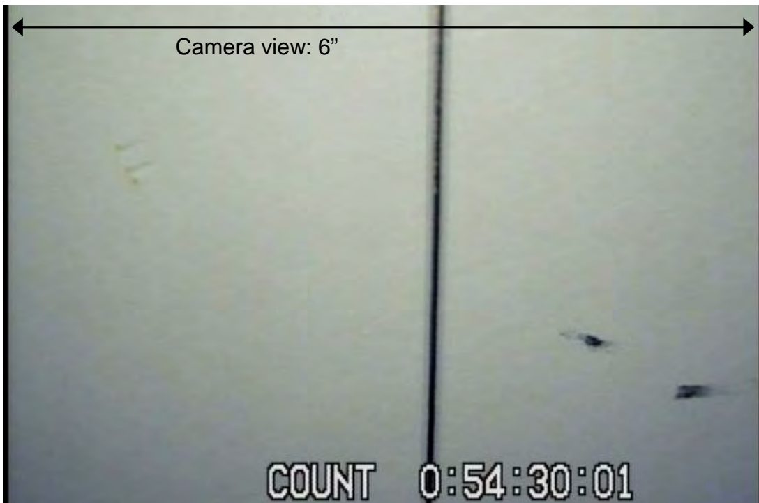
29. Scan 30 slight rust discoloration and black stains
