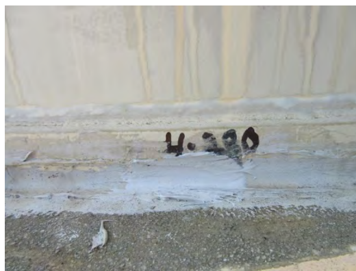
18. Cell 4 Caulking As-Left
