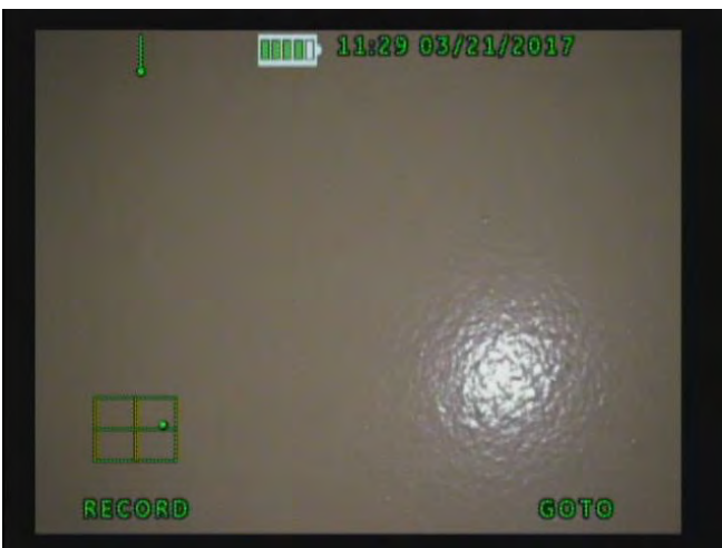
12. Close-up of overpack coating
