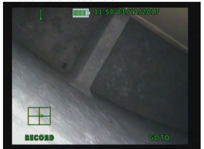
6. Vault Liner and Seismic Shim
