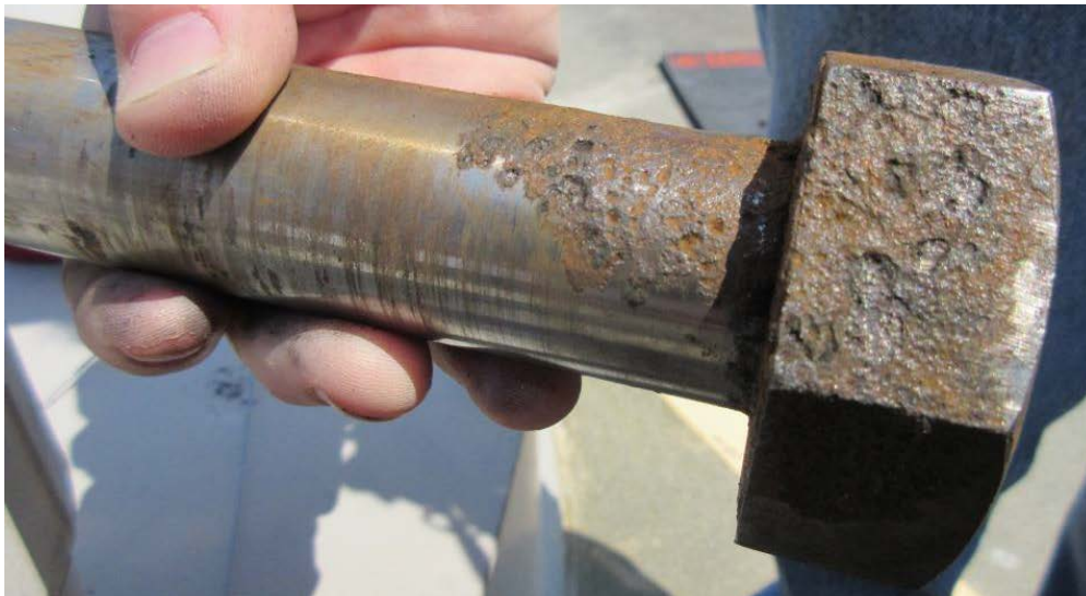
66. Removed bolt following cleaning (pitted bolts replaced)
