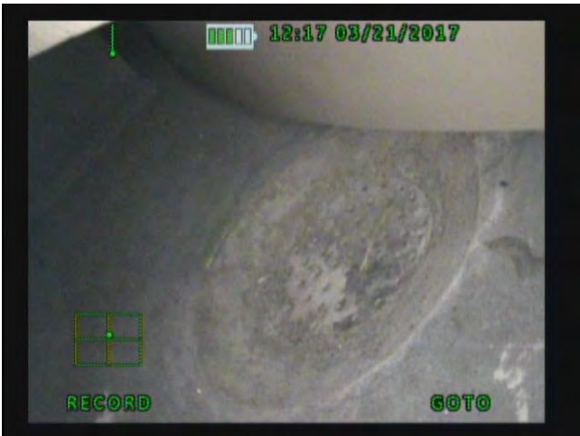
5. Vault Liner Bottom and Vault Drain
