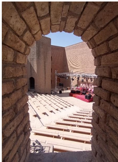
Figure 7. Open Theatre in Erbil Citadel, photo by the (Author).
