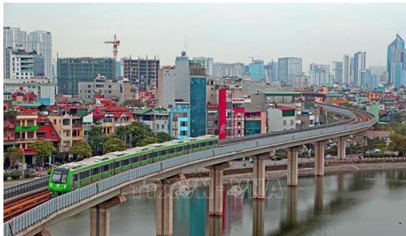
Fig. 3 – Cat Linh-Ha Dong railway bridge
