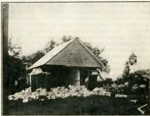
King's Gate Chapel, Jamaica, after the earthquake.
