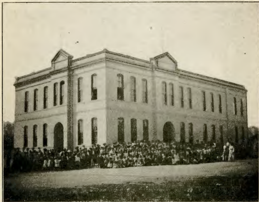
Mission Building, Monterrey, Mexico.
