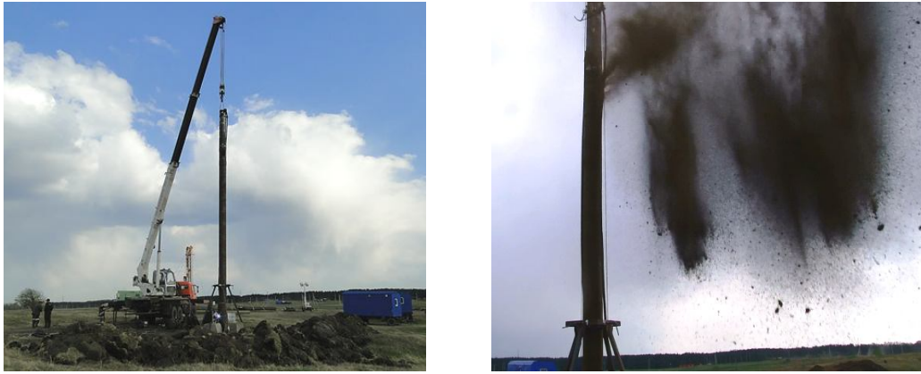
Fig.3. Application of technology for installation of starting conductors
