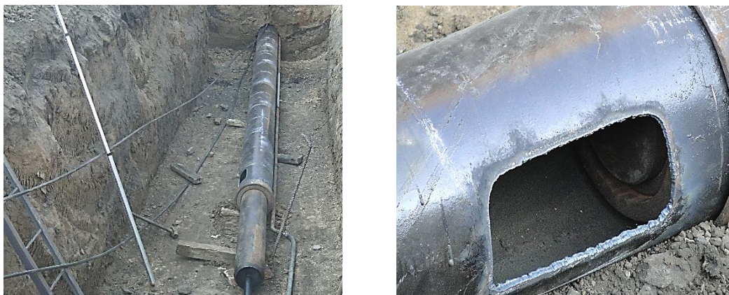
Fig.4. Application of technology for trenchless laying of communications
