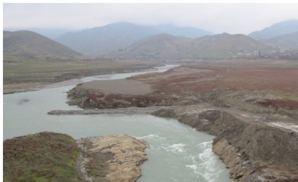
Fig. 1. View of the flood gorge from the dam of the Mataghis Reservoir. A river bed formed in the accumulated sediments due to hydraulic flushing
