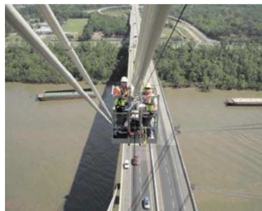
Fig 2. Cable inspection with hanging lift.
