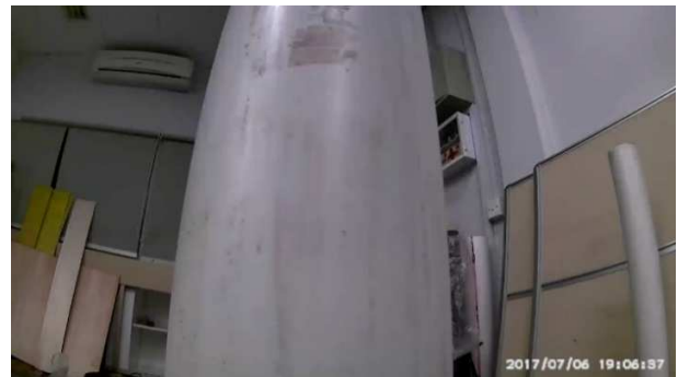
Fig 9. Captured inspection image from camera
