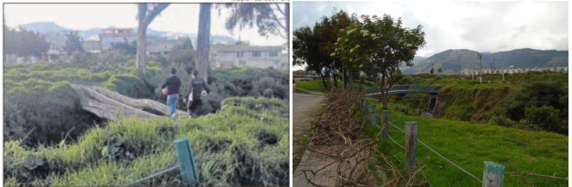
Figure 6.11. On the left, an improvised bridge between Ciudadela del Ejército and Ciudadela Ibarra (Últimas Noticias, 2013). On the right, a bridge (built years later) 30 metres away from the first to cross ravine Calicanto .
