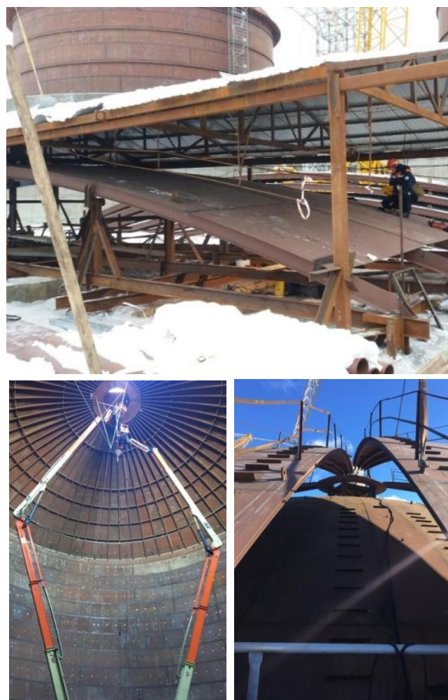
Figure 3. Sheet prefabrication and roof installation on a tank.
