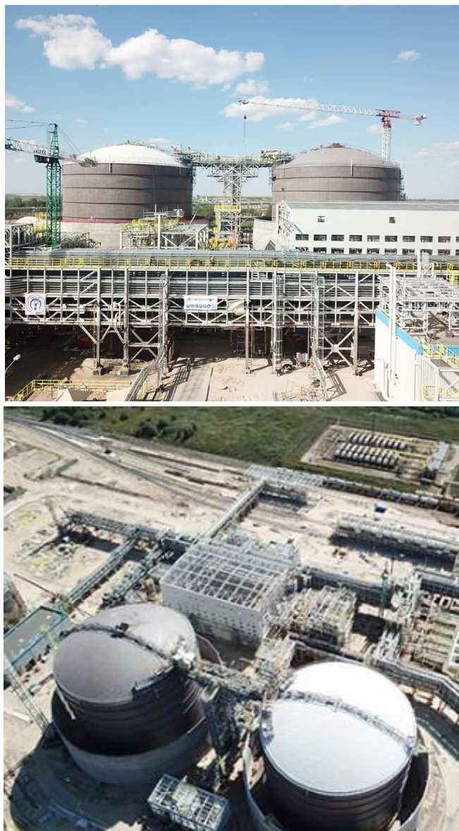
Figure 1. The Kingisepp plant; appearance of two ammonia storage tanks with double walls.
