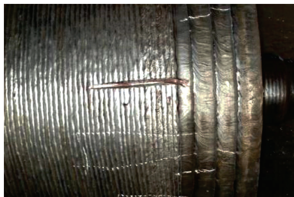
Cracks in field F
