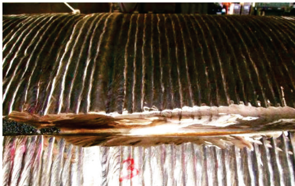
Cracks in field D
