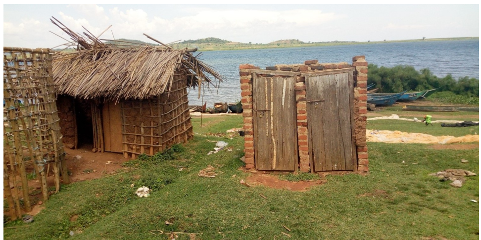
Fig 3. Examples of pit latrines in the studied communities.
