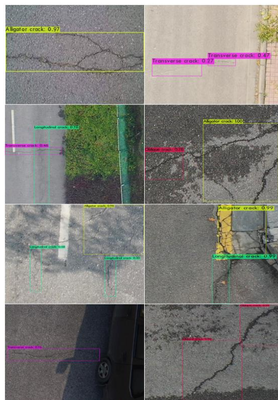
Figure 5. Some samples of pavement distress recognition results using proposed deep learning network.
