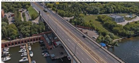
Direction from E to D (Strogino Bridge and Novoshchukinskaya Street)
