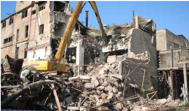
Fig. 1. Typical construction site (dismantling - construction)
