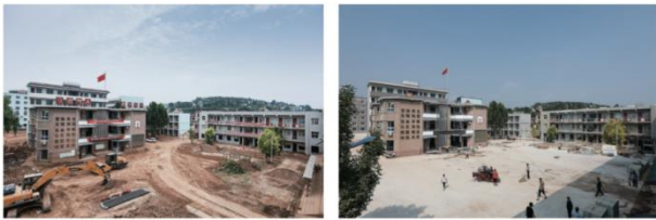
Figure 4. Left: Before the renovation of the No. 1 Junior High School in Kangdian Town, Gongyi City, Henan Province. / Right: After repair [7].
