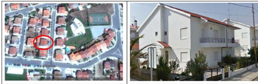
Fig. 2. Location and facade of the building.
