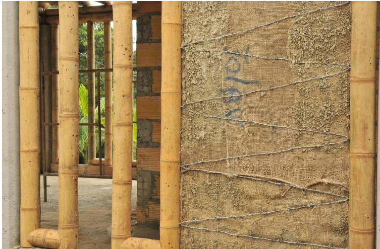
I.66 The panel (from Archdaily Bahareque, a seismic resistant construction technique in Colombia) / Il pannello / El panel
