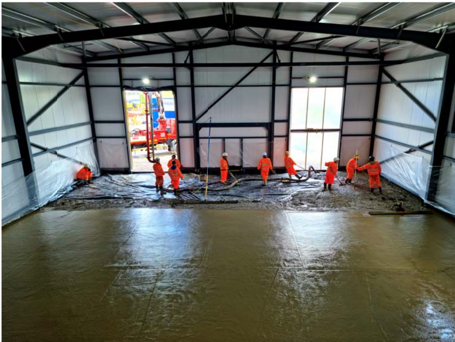
241 Figure 4: Solstice Park development; slab pour underway
