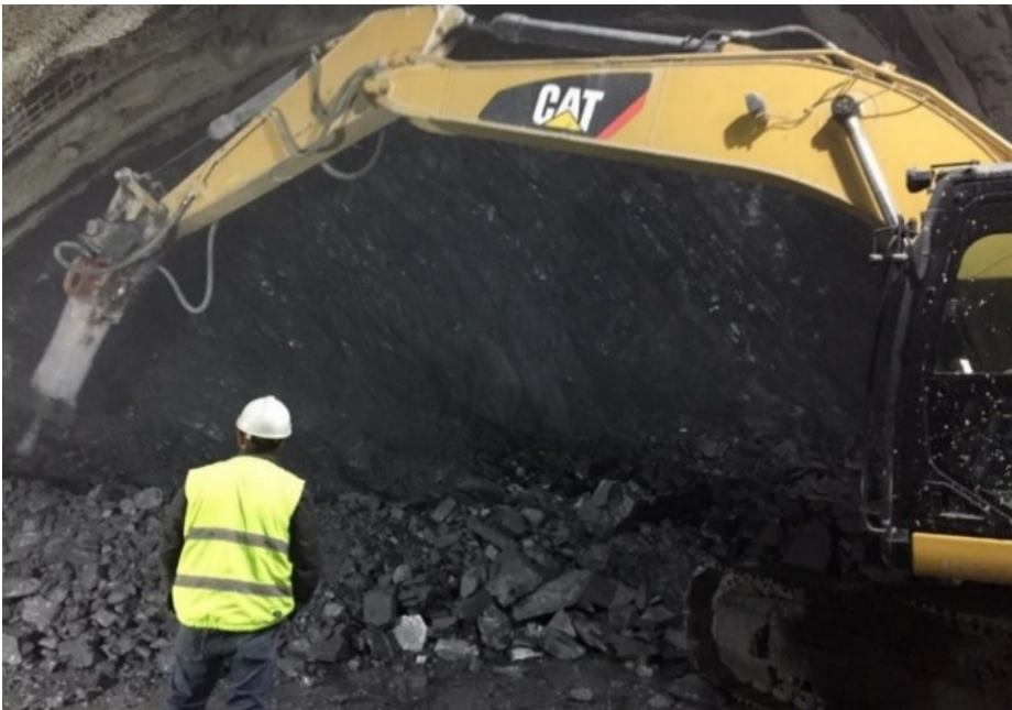
Figure 3-1: System used to excavate Uskudar-Cekmekoy tunnel
