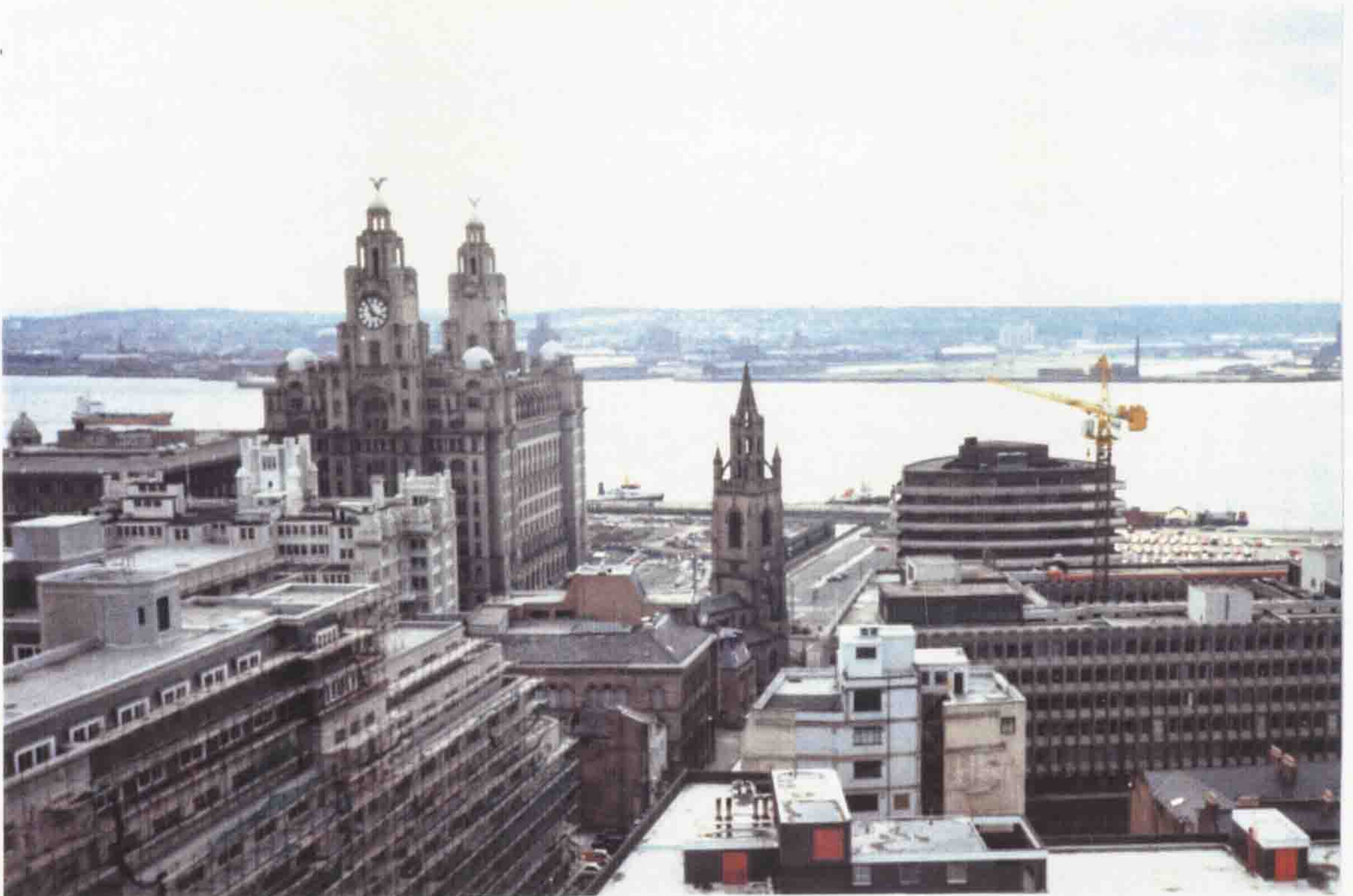
Plate 4.2 Photograph taken from the roof of the building looking southwards and across the River Mersey.
