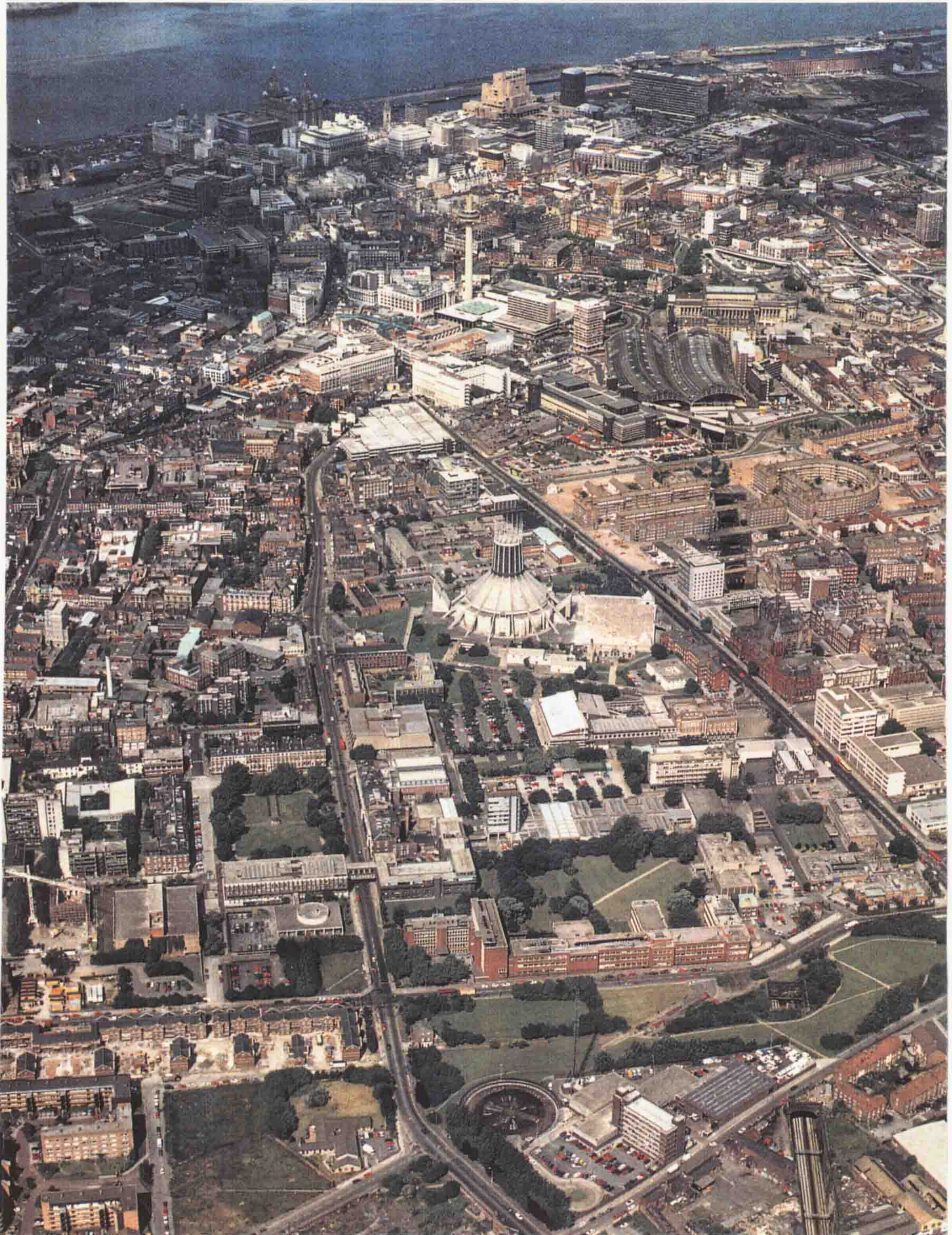
Plate 4.5 Aerial photograph of Liverpool city centre and the surroundings.
