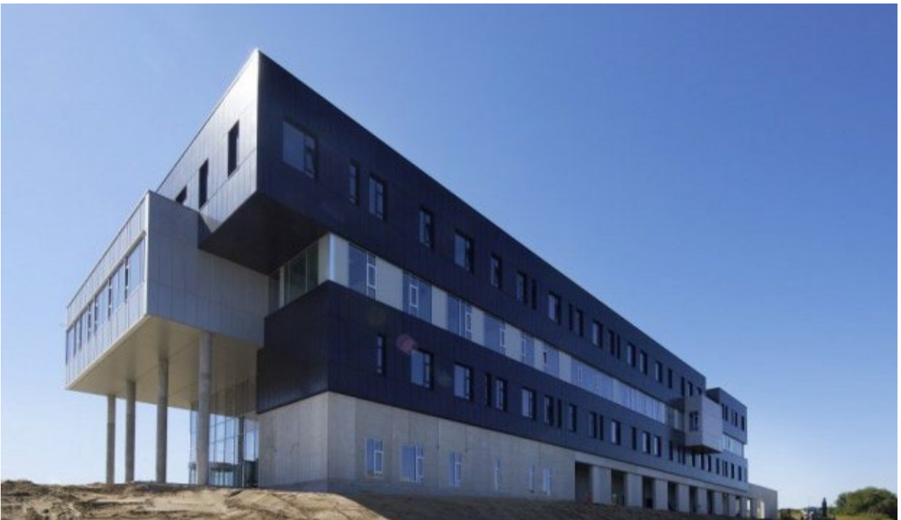
Figure 8: View of the North facade of the TMV 23 building.
