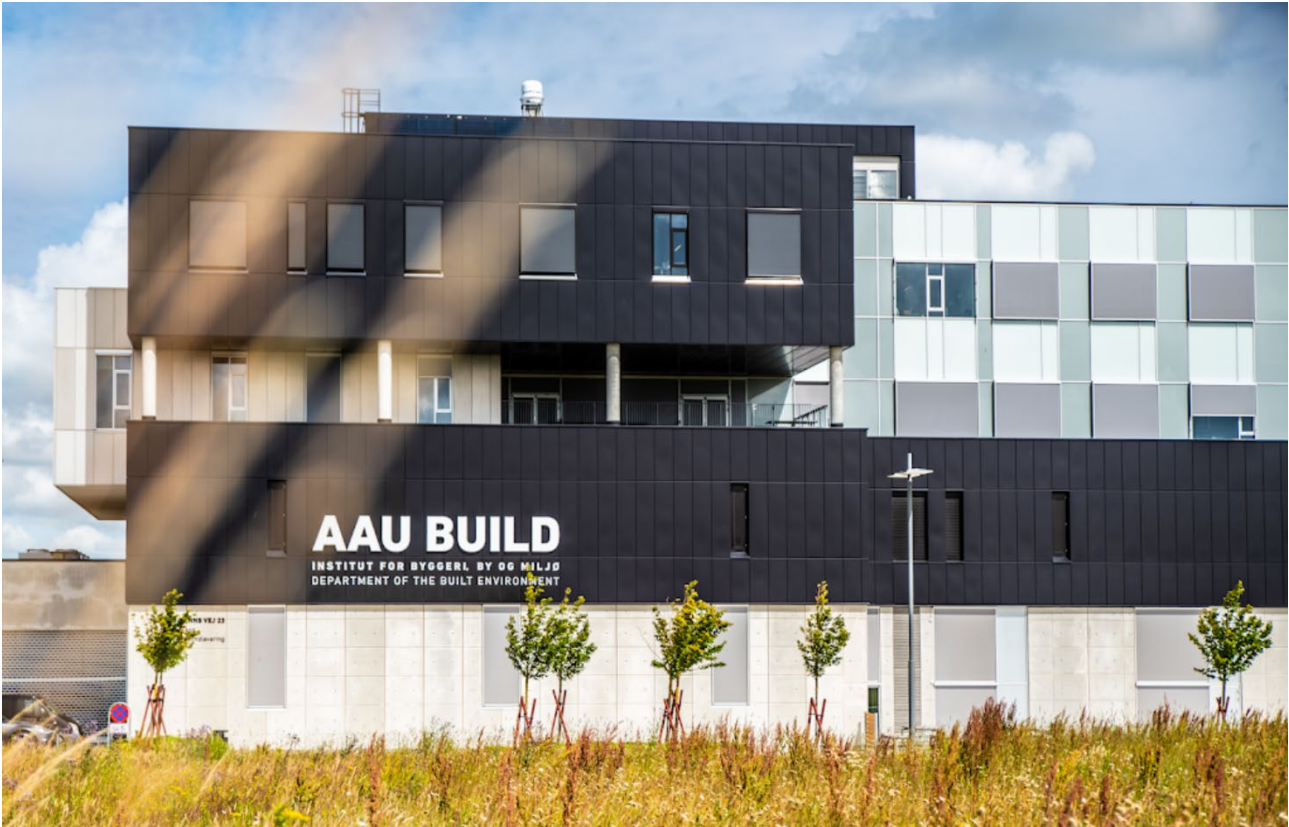
Figure 5: View of the South facade of the TMV 23 building (credit to Aalborg University).
