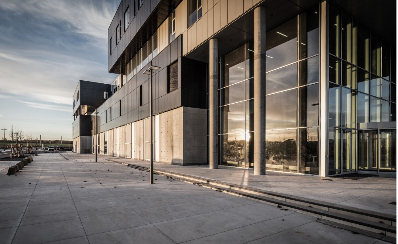
Figure 7: View of the South facade of the TMV 23 building (credit to Ronge Fotografi).
