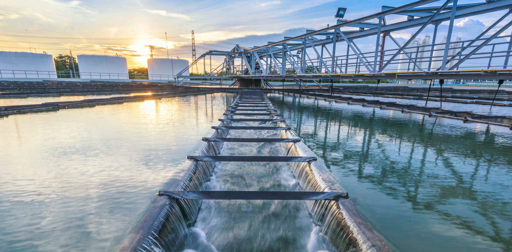
Image caption: Water holding pools at a drinking water plant. Photo from iStock.
