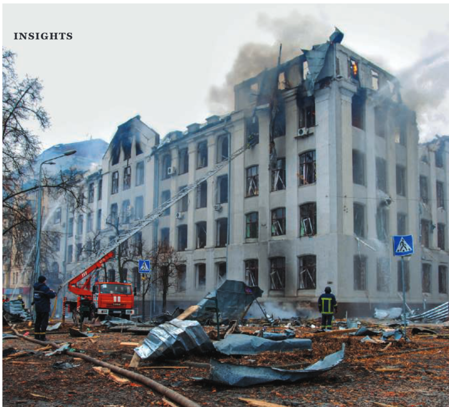
Russian shelling damaged this Kharkiv National University building in March 2022. As Russia's invasion continues, scientists who remain in Ukraine would benefit from international support and remote opportunities.
