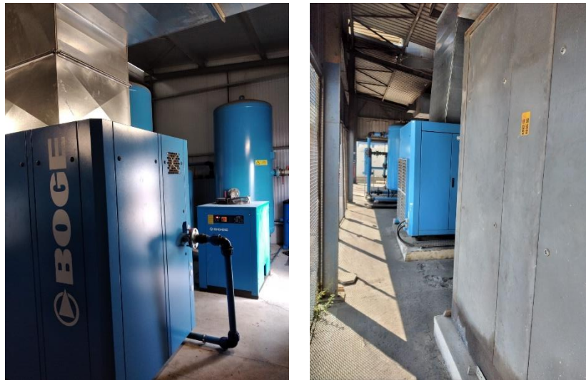
Figure 23: Production of Compressed Air
