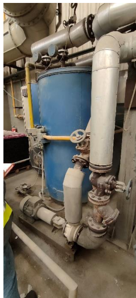
Figure 25: Thermal oil Boiler
