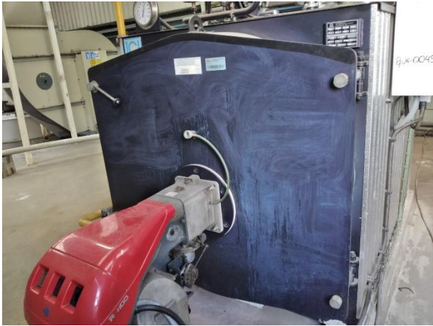
Figure 24: Boilers of hot water
