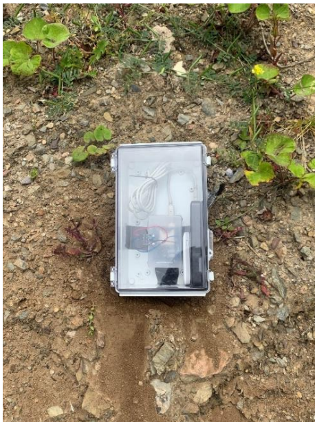
Figure 4. 39 Sensor deployment on Connolly Street slope, Cobh
