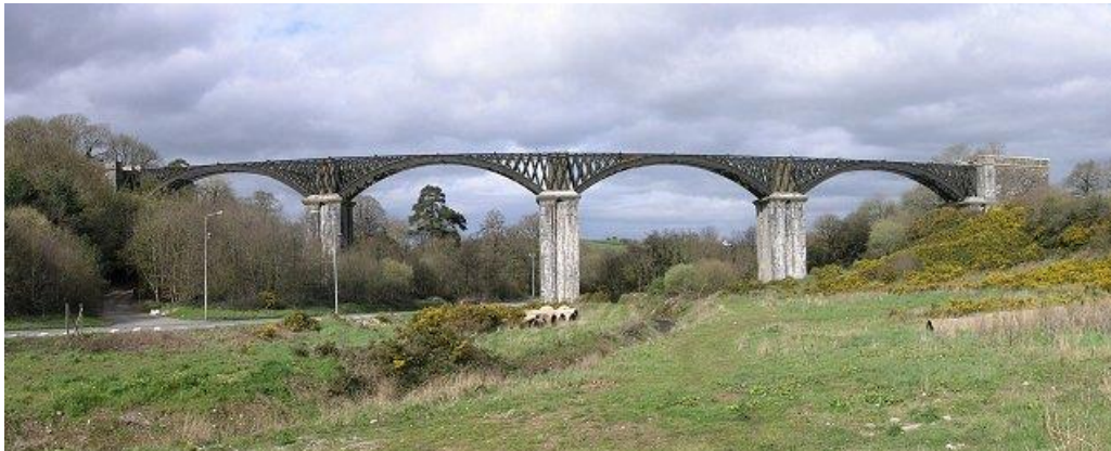
Figure 3. 16 Chetwynd Viaduct, Cork previously subject to laser scanning technology (15)
