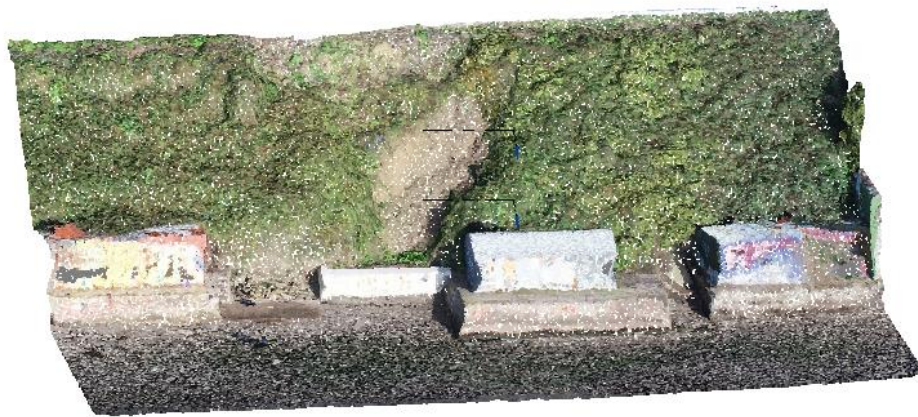
Figure 5. 14 Point Cloud of Connolly St. slope in Revit
