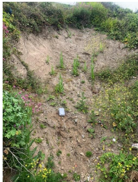
Figure 4. 38 Sensor deployment on Connolly Street slope, Cobh
