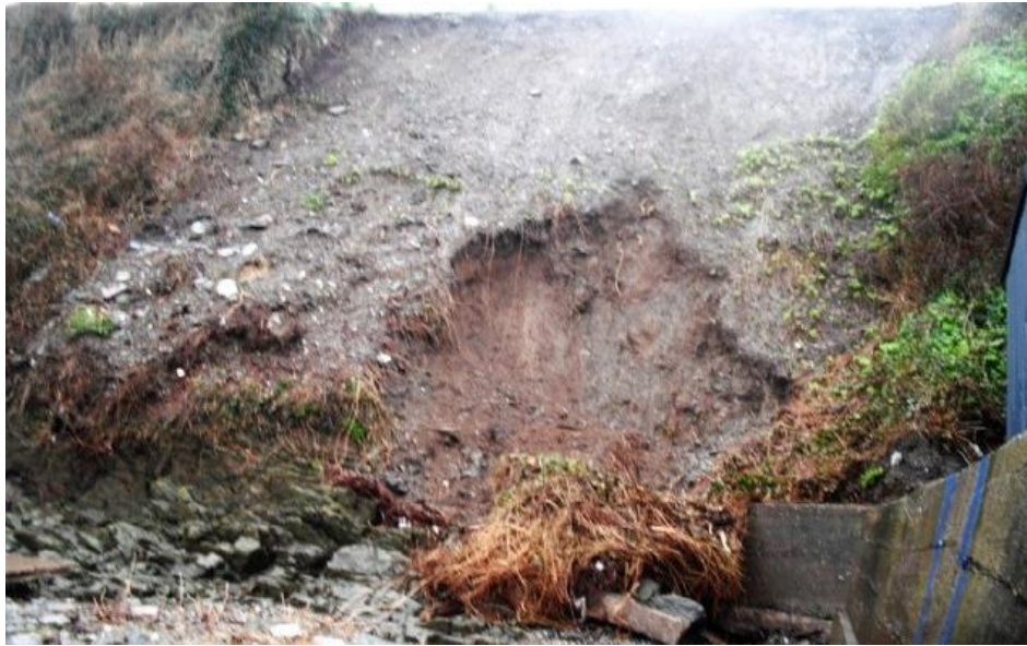
Figure 1. 2 showcases a section of further partial landslide on the Connolly Street slope (1)
