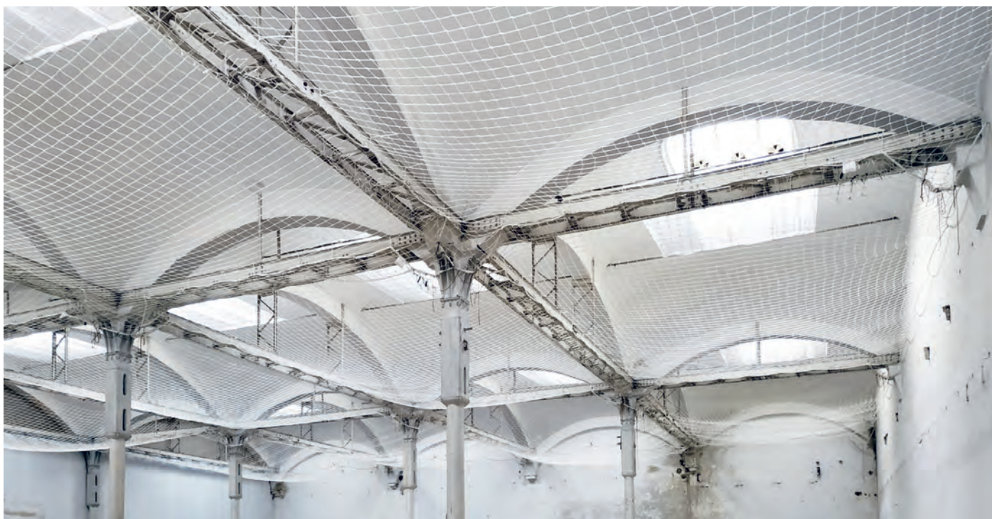
Interior de Can Bagaria (Fuente: Martín E., 2019) / Can Bagaria interior (Source: Martín E., 2019)
