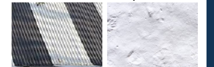
Corrugated iron roofs
