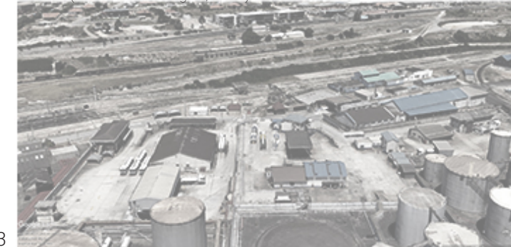
Figure 081: Manganese Tank Site Warehouses Source: (Maxer Technologies, 2020)
