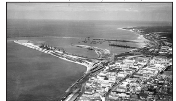
Figure 064: Harbour History in 1936. Source: (Port Elizabeth | The Heritage Portal, 2020)
