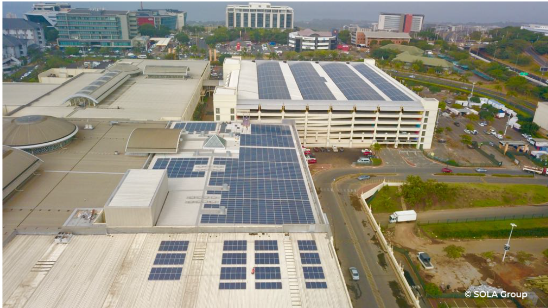
Photo 7.1 Flat mounted panels at Gateway Mall, KZN
