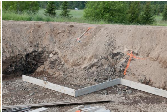
Figure 5b. The excavation of soils for our foundation.
