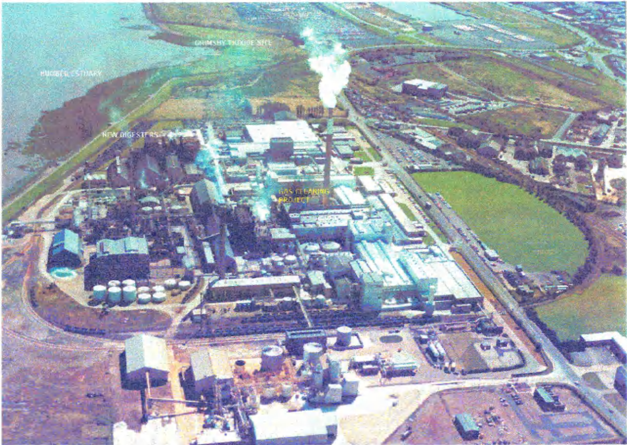
P10 Scanned aerial photograph of Tioxide Grimsby site
