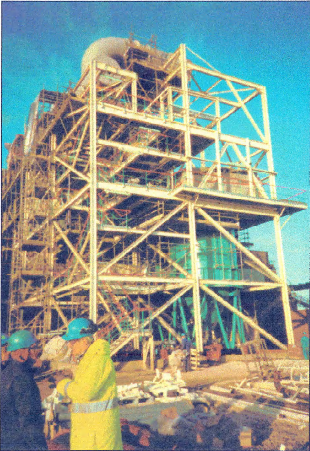
P 05 Photograph of New Digester project (Project 2)
