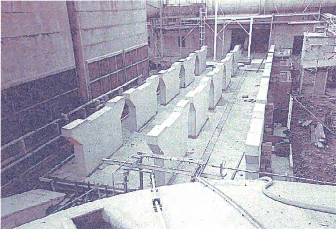
P03 Photograph of civil plinths under construction (Project 1)
