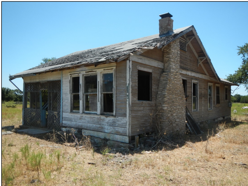
Figure 15. View of the north and west facades of Structure 5, facing southeast.
