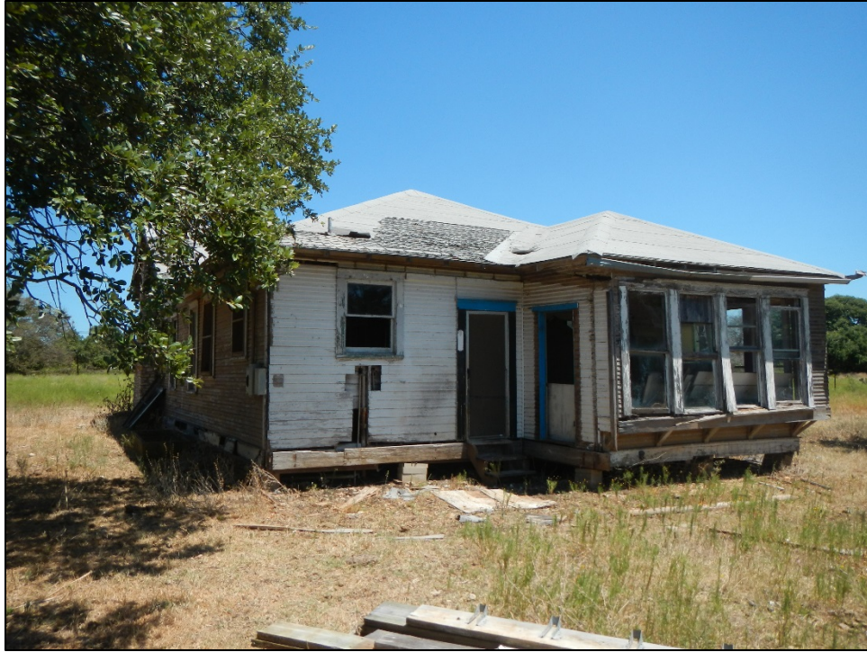
Figure 14. View of the south elevation of Structure 5; facing north
