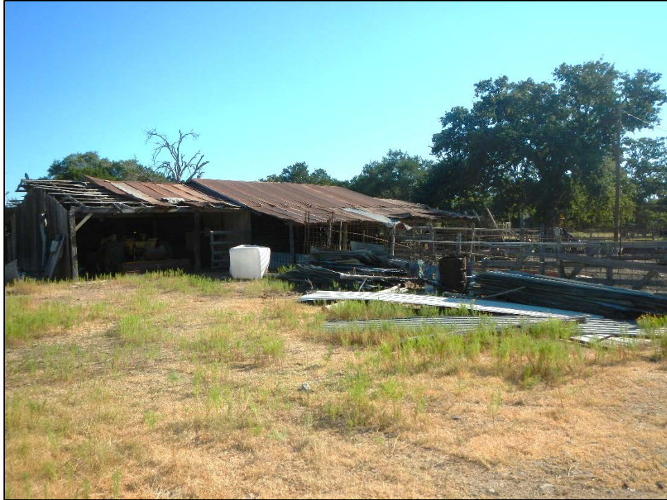
Figure 23. Overview of Structure 3 at site 41WM1343; facing northeast.
