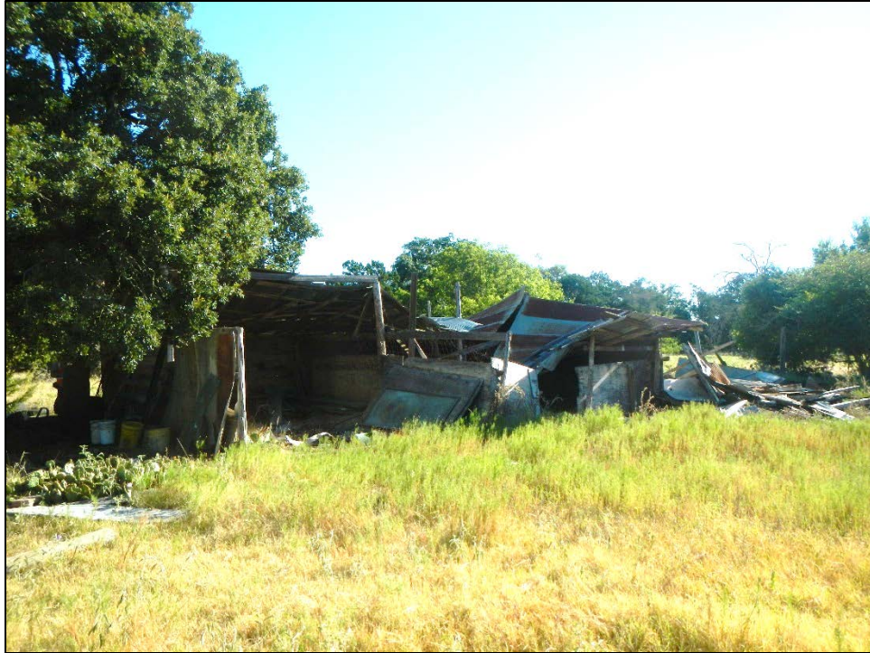
Figure 21. Overview of Structure 1 at site 41WM1343; facing northeast.
