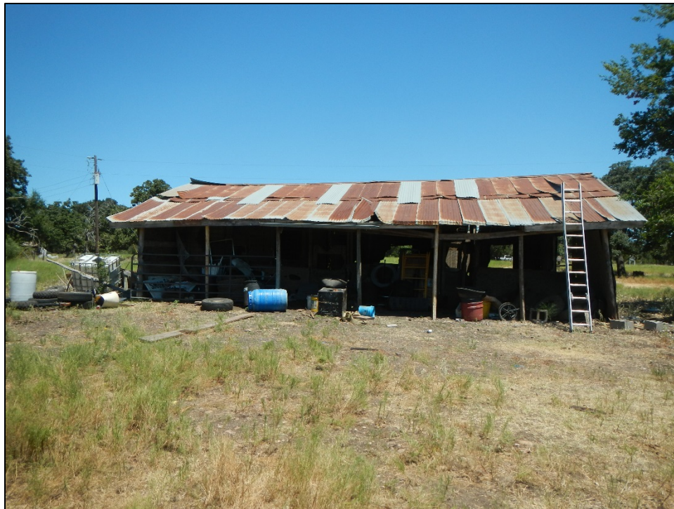
Figure 11. East view of Structure 4 at site 41WM1342; facing west.
