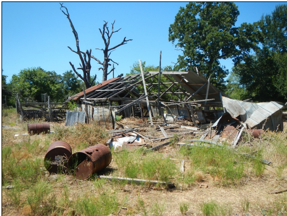
Figure 7. Overview of Structure 1 at 41WM1342; facing southwest.
