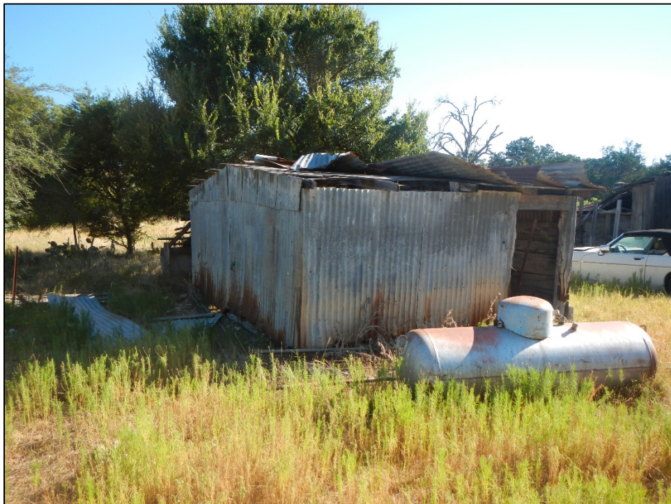
Figure 22. Overview of Structure 2 at site 41WM1343; facing northeast.
