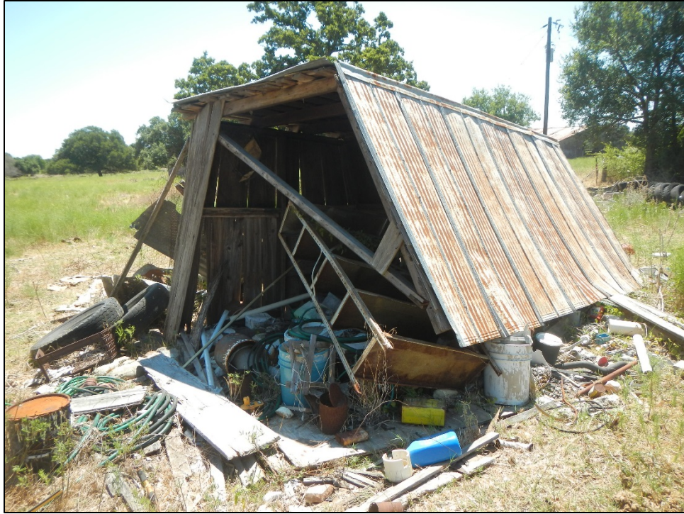
Figure 9. Overview of Structure 3 at site 41WM1342; facing east.
