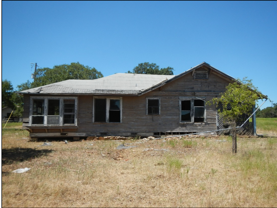
Figure 12. Overview of Structure 5 at site 41WM1342; facing east.
