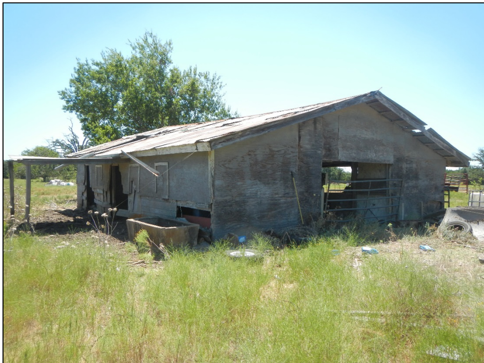
Figure 10. Overview of Structure 4 at site 41WM1342; facing northeast.
