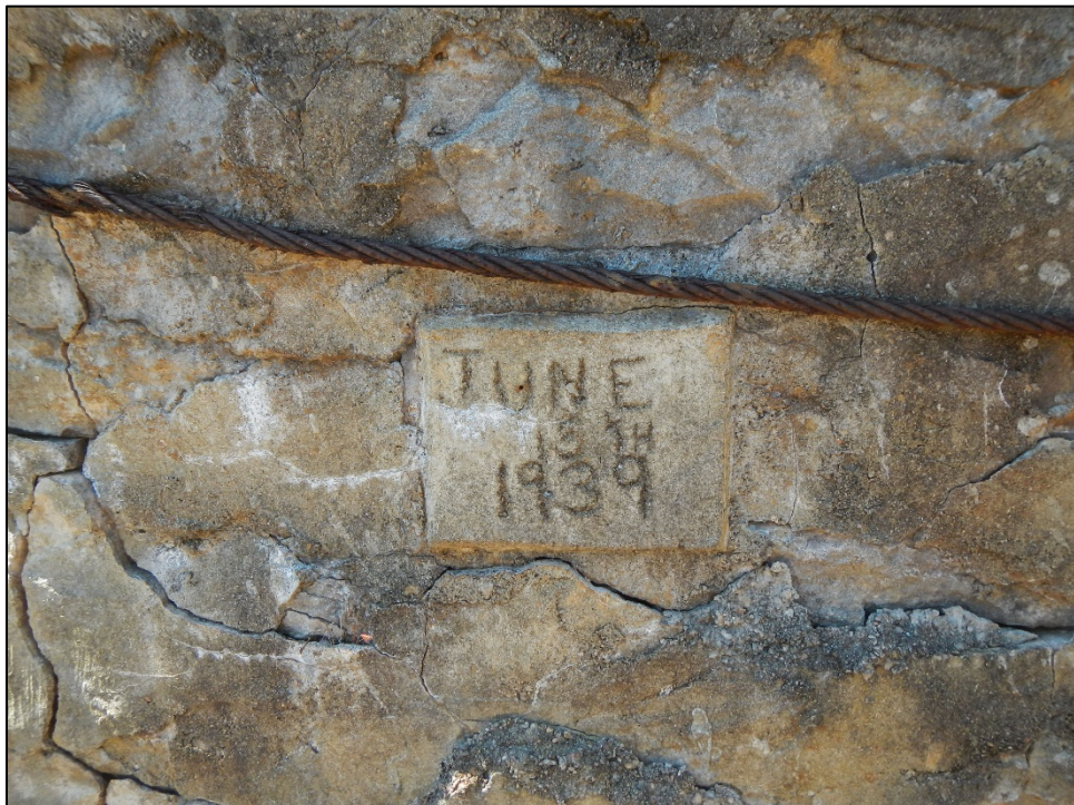
Figure 17. Plaster plaque that has been etched with "JUNE 15 th 1939"; facing south.
