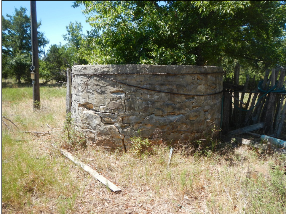
Figure 16. Cistern at site 41WM1342; facing south.
