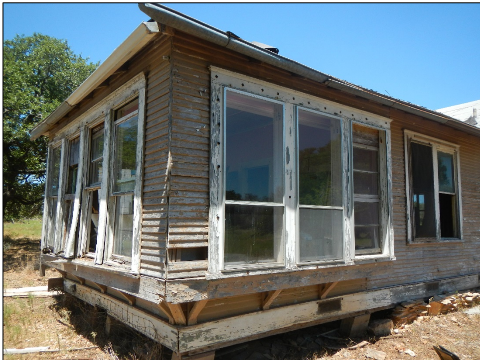
Figure 13. View of the foundation of Structure 5 at site 41WM1342; facing west.
